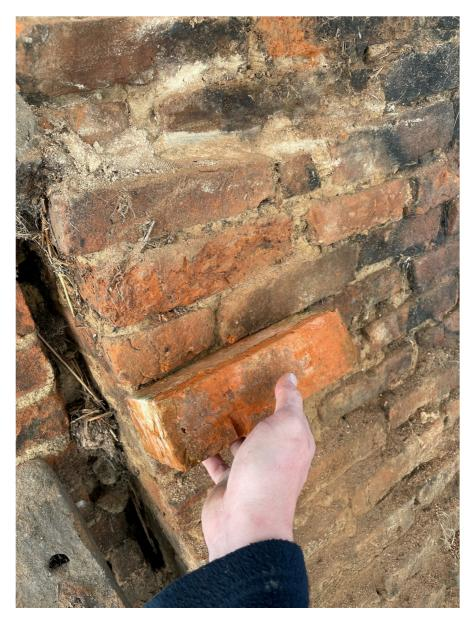
The existing chimney bond is a mixture of lateral bond at low level forming a traditional stretcher bond at high level. The proposed brick bond at high level will be a traditional stretcher bond to match existing with the bricks laid in a mortar mix consisting of a 3 part sharp sand to 1 part NHL 2. The render will not be reintroduced to the top section of the chimney as existing, with reclaimed brick in a traditional stretcher bond visible.
