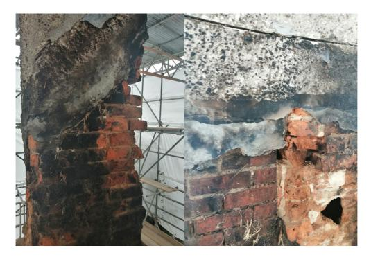
Works commenced on the property in association with the granted applications. However, the chimney stack is in far worse condition than was anticipated at the time of the original applications and the loss of brick section around the original chimney at roof line requires this area to be completely rebuilt. With loss both internally and externally and a number of holes all the way through, and do not consider we can carry out an effective repair safely in its condition.
