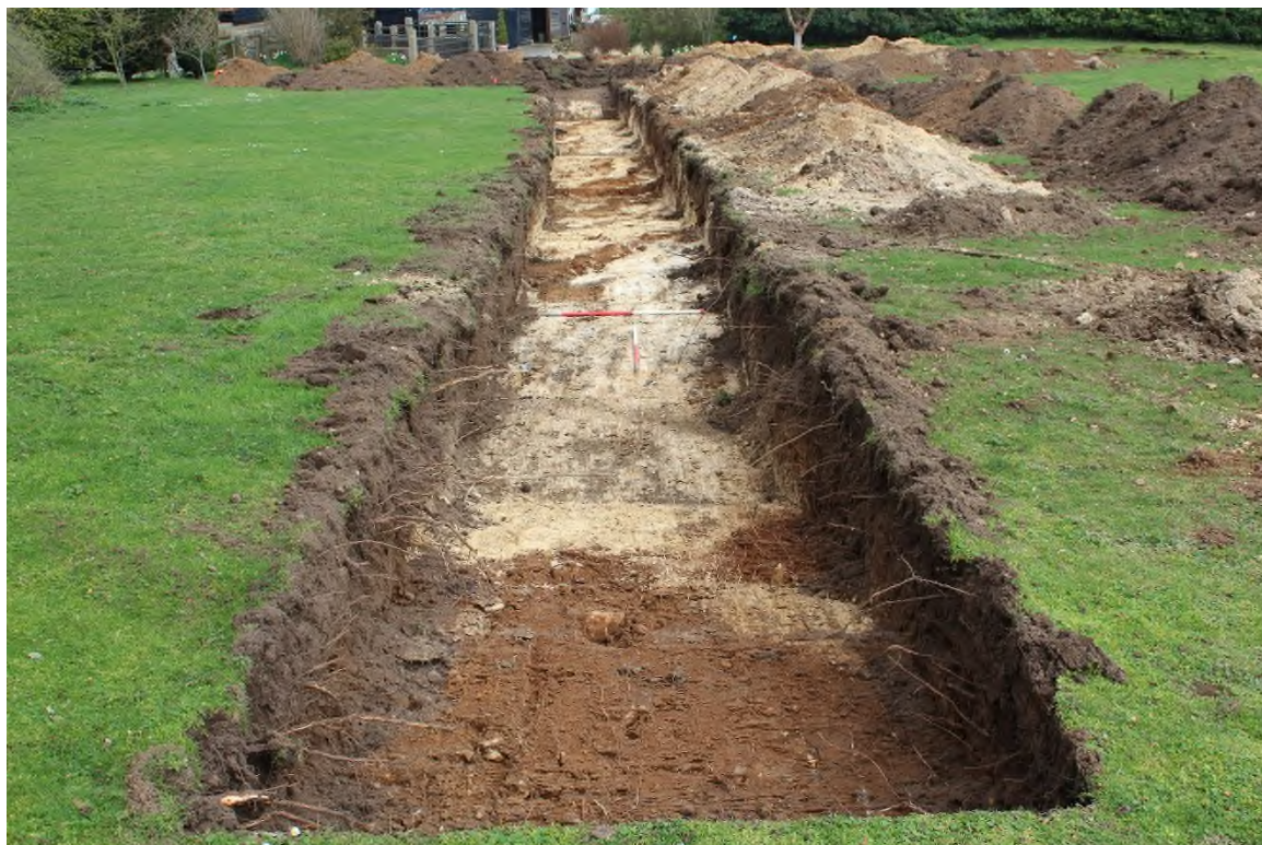
Plate 8: Trench 6, looking northeast
