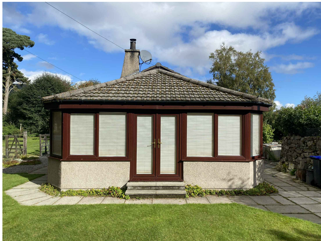
SIDE VIEW OF THE EXISTING SOMERSET COTTAGE SUN LOUNGE
