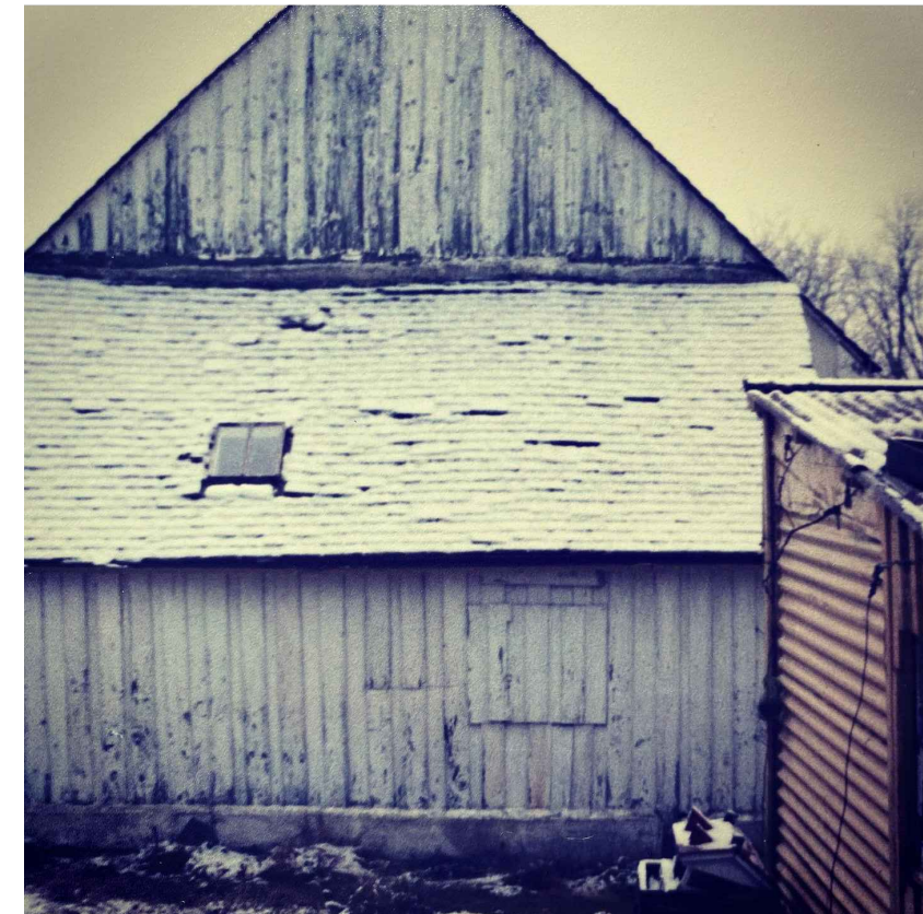
HISTORIC PHOTOGRAPH OF THE ORIGINAL 25 MAR ROAD COTTAGE, WHICH WAS DEMOLISHED TO MAKE WAY FOR THE CURRENT SOMERSET COTTAGE
