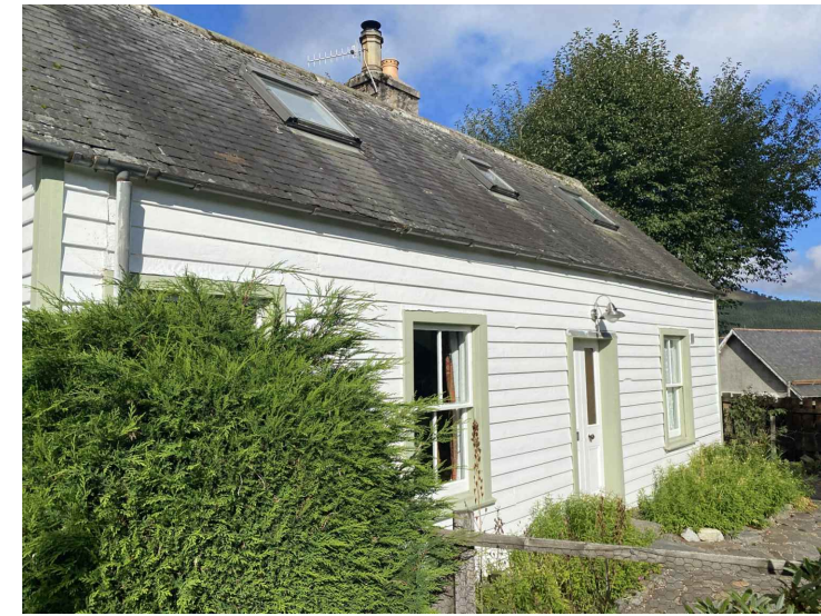
THORNBANK VIEW 3 - BESIDE SOMERSET COTTAGE
