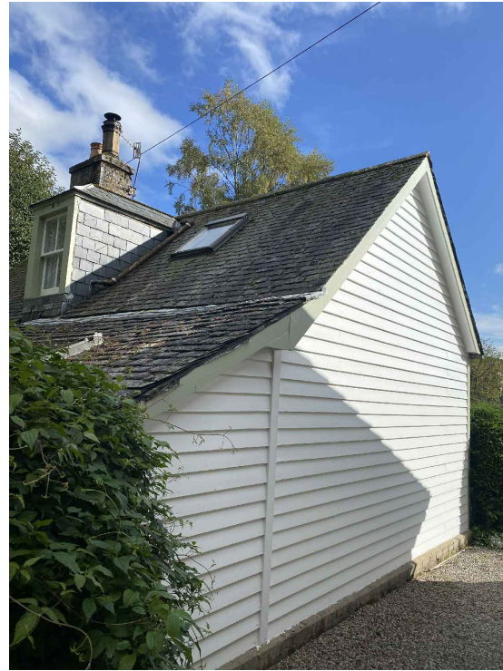
THORNBANK VIEW 2 - BESIDE SOMERSET COTTAGE
