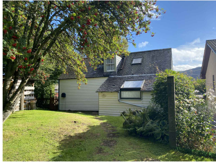
THORNBANK VIEW 1 - BESIDE SOMERSET COTTAGE
