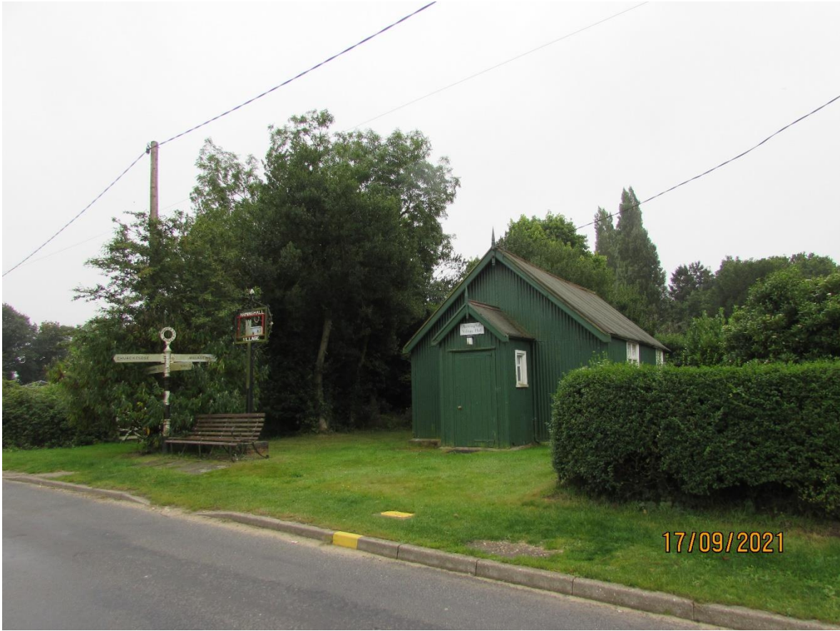
Overview of site from road looking south east
