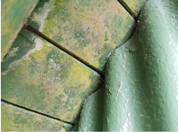
Photo 7: Corrugated metal wall finishing flush with roof at gable end
