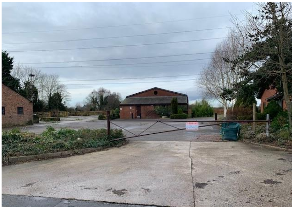
View into former Hultons site with south-western facing elevation of office building located to the right of photograph
