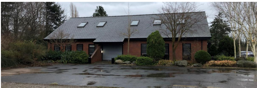
Fig 2: View of existing office building
