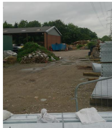
Fig 8: Area of hard surface formerly used for storage of materials
