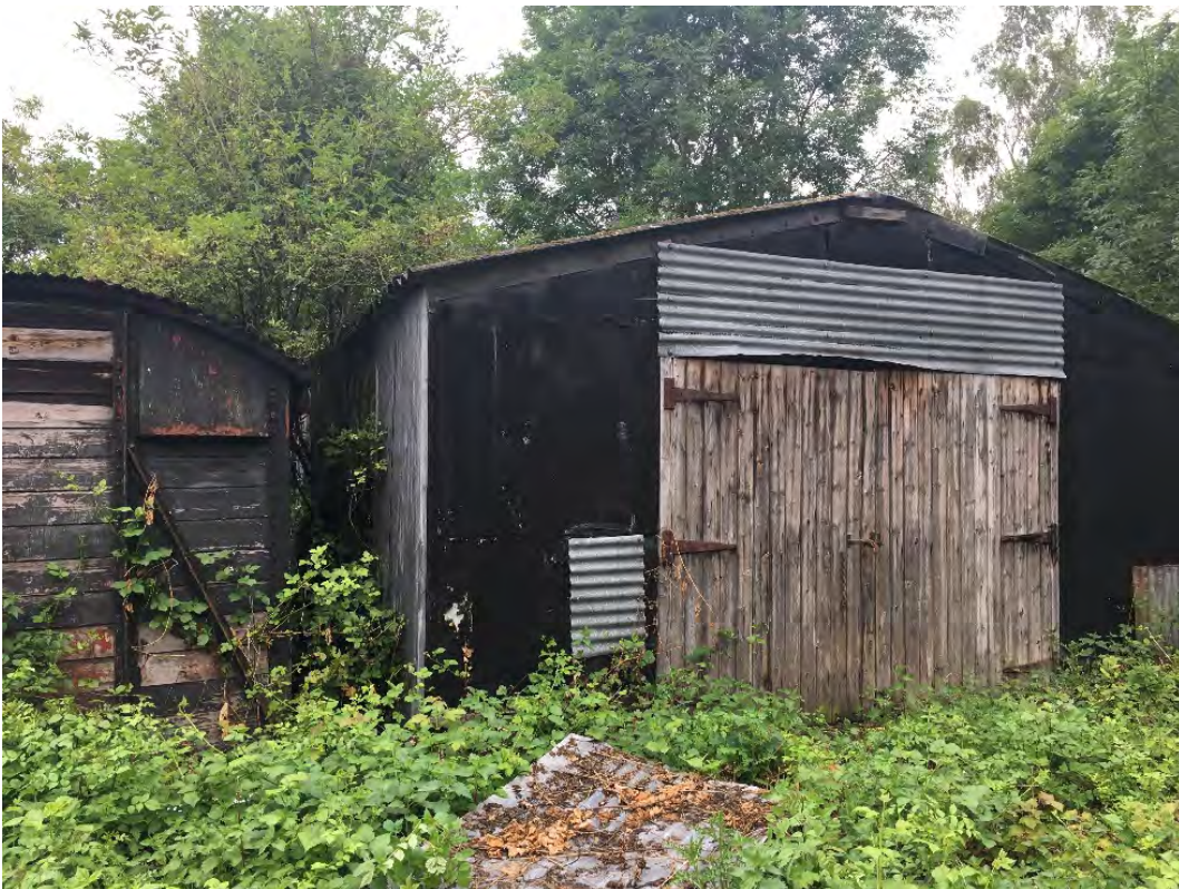
Photograph 14 – Buildings 11 (left) and 12 (right)
