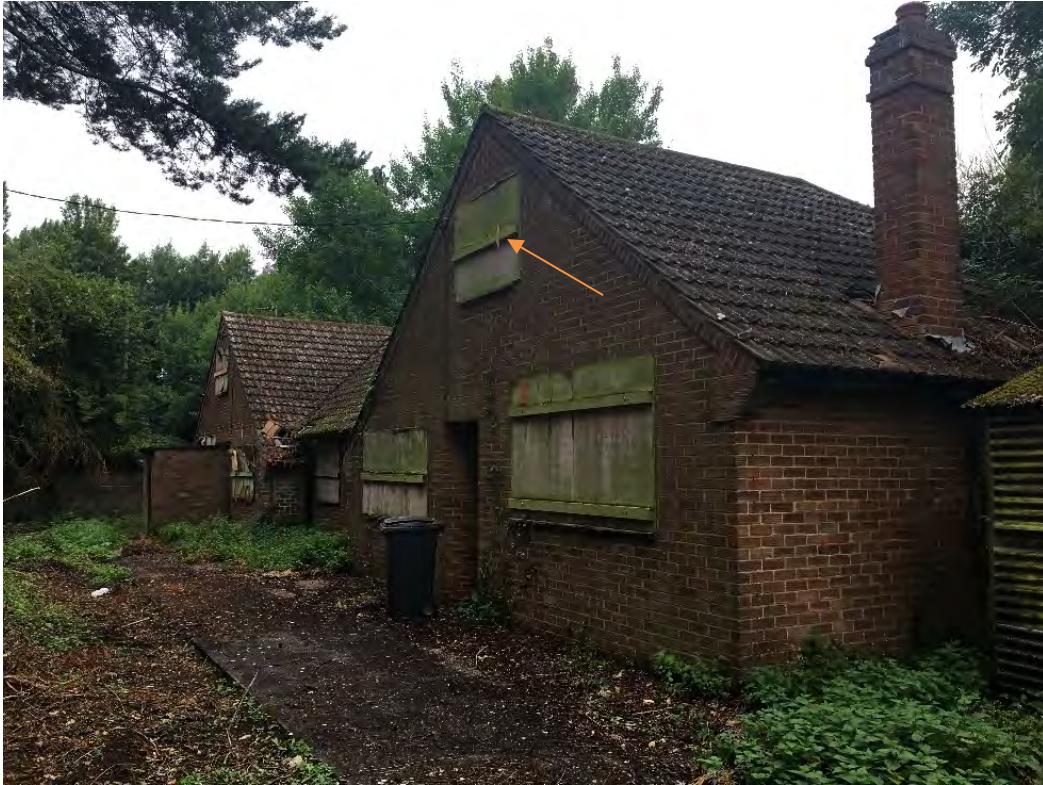
Photograph 5 – Western aspect of Building 1 with roost location behind wooden boarding
