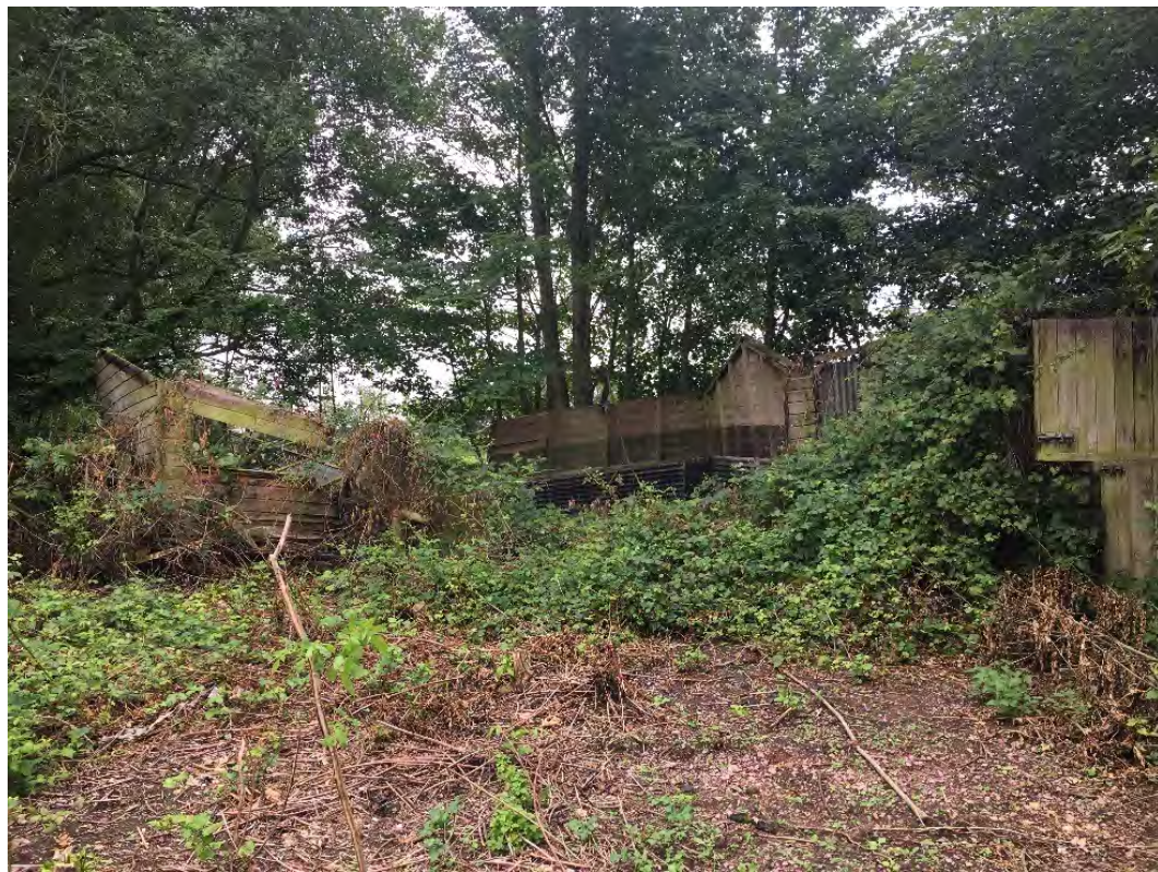
Photograph 12 – Building 9a and b
