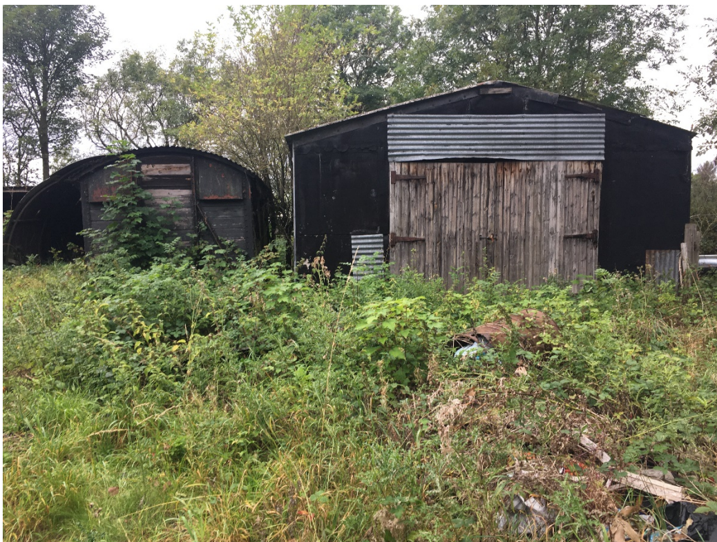
Plate 2: View towards some of the outbuildings within the western extent of the site
