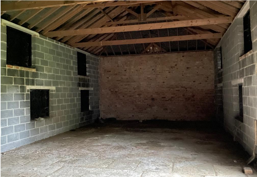
Photograph 6: Internal view of Building 2
