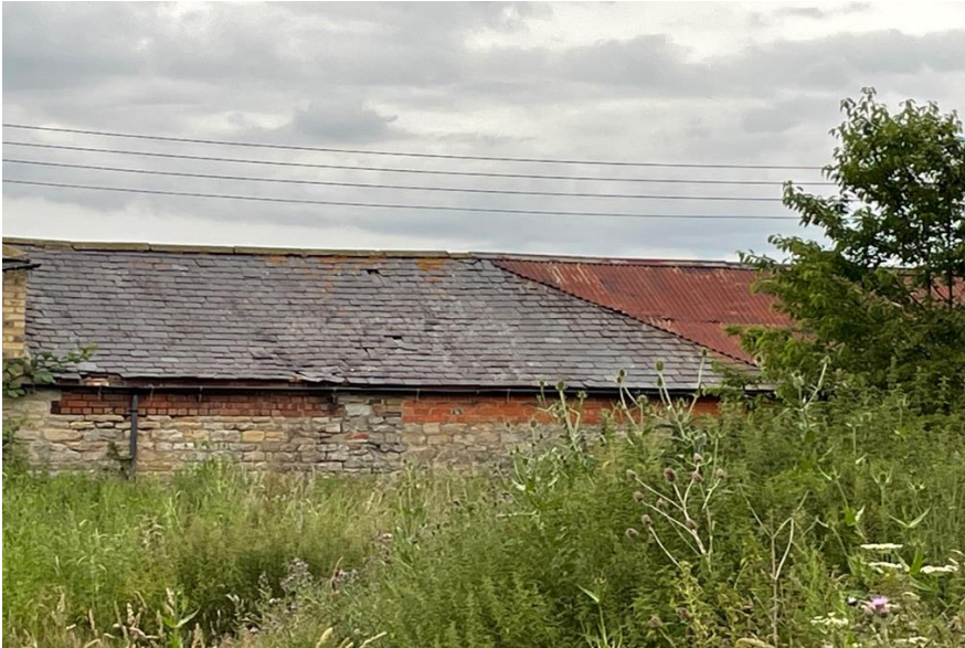
Photograph 2: Building 1 - southern elevation
