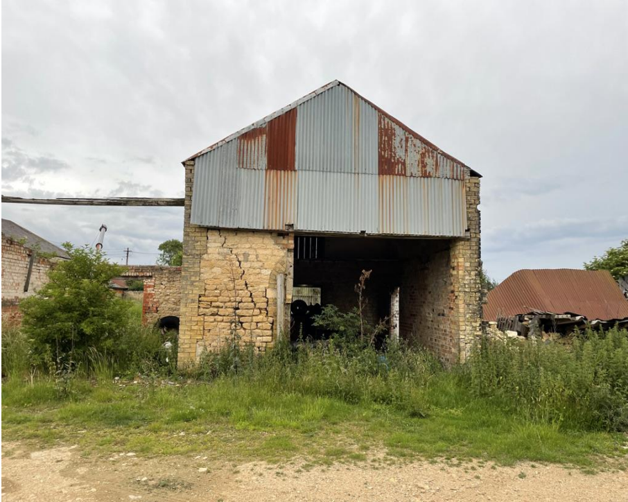
Photograph 10: Building 3 - western elevation
