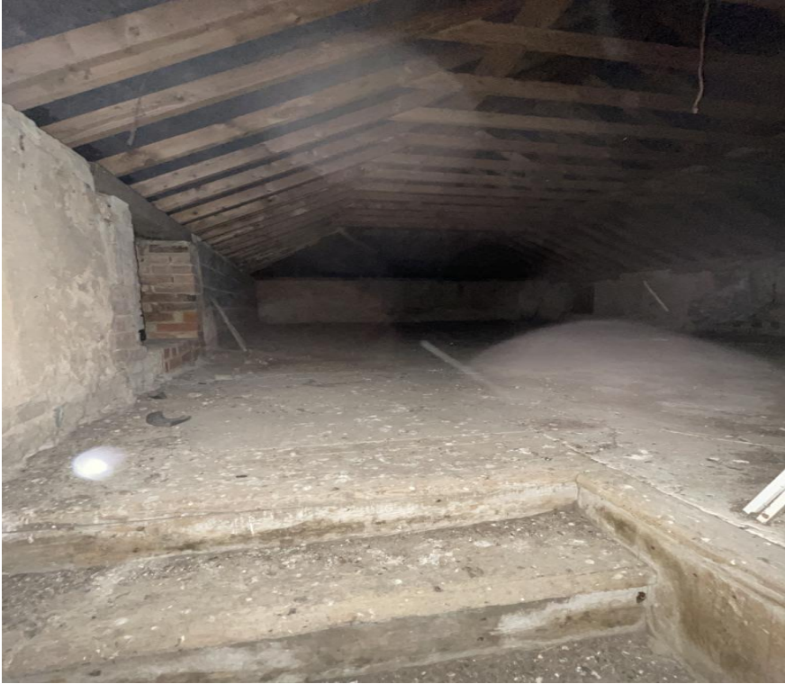
Photograph 7: Upper floor of Building 2
