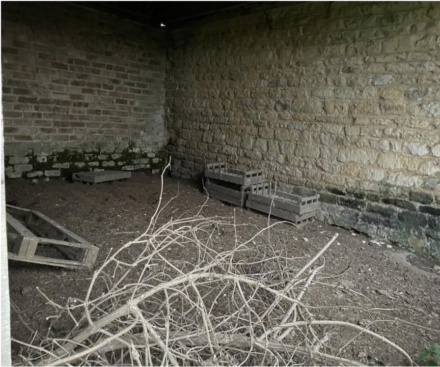
Photograph 9: Further view of lower floor area of Building 2
