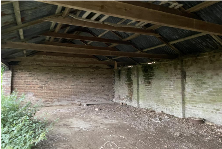
Photograph 3: Internal view of Building 1
