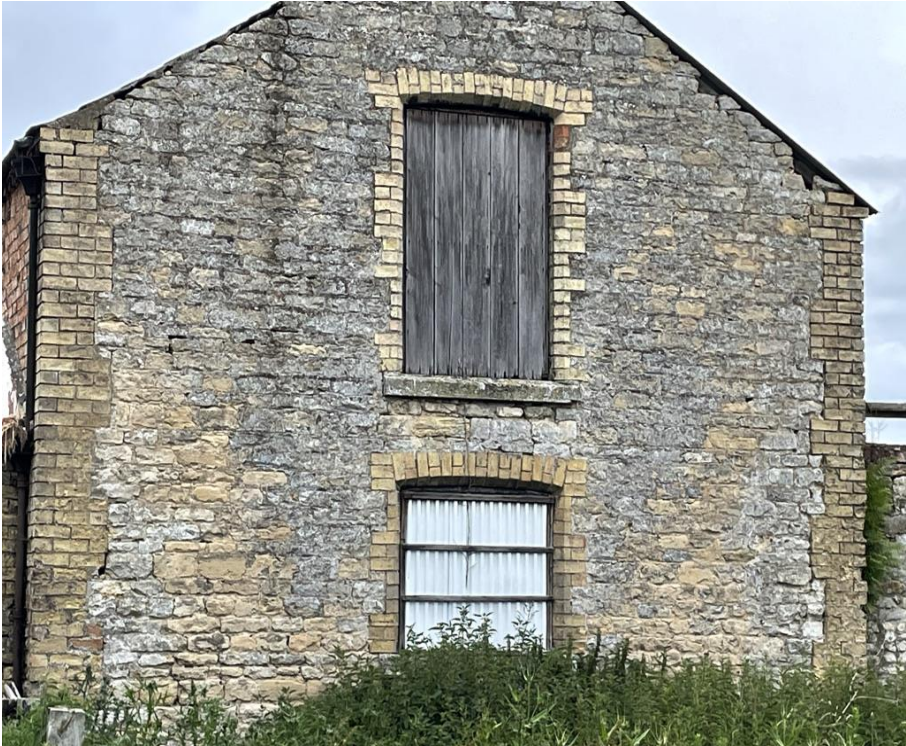
Photograph 11: Building 3 - eastern elevation
