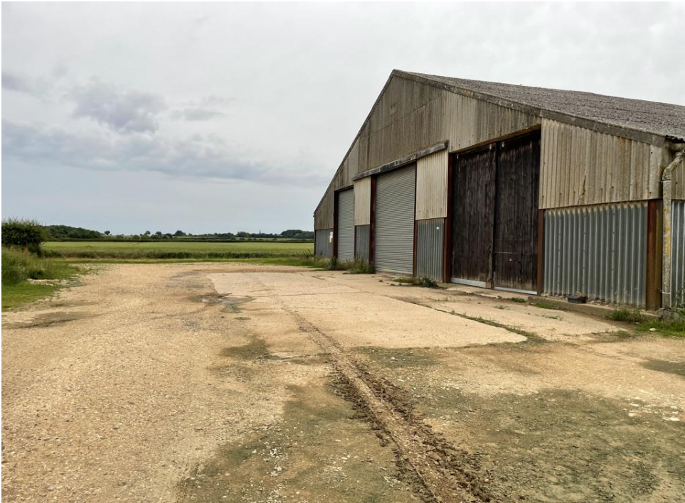
Photograph 14: Farm building located to the west
