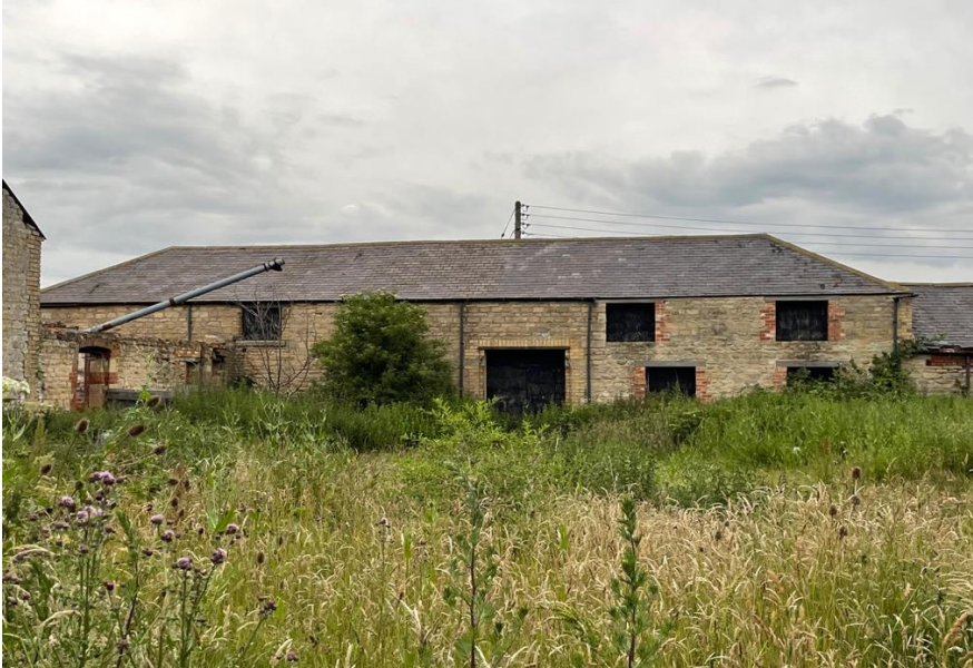
Photograph 5: Building 2 - southern elevation
