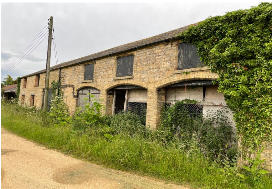
Photograph 4: Building 2 - northern elevation
