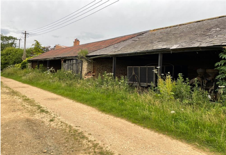
Photograph 1: Building 1 - northern elevation
