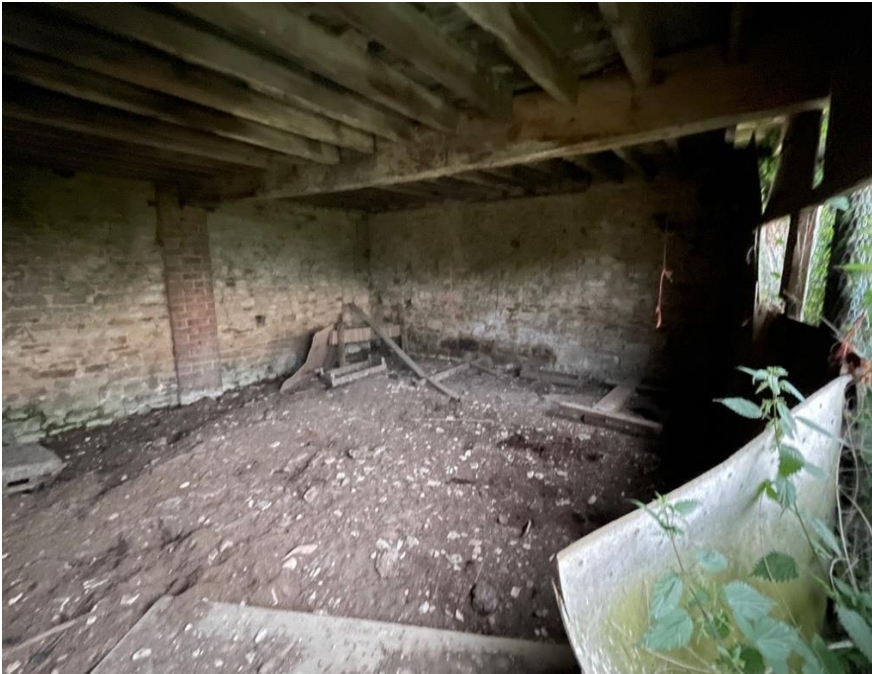
Photograph 8: Lower floor area of Building 2
