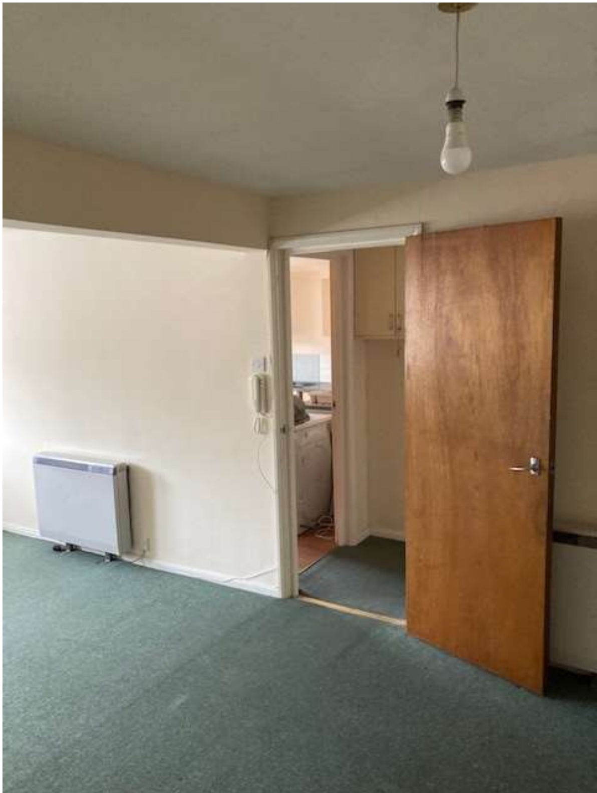
Figure 10: Partition between present kitchen and living room for removal
