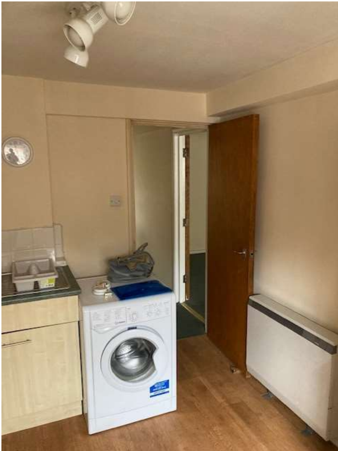
Figure 12: Present kitchen door to be blocked and cupboard inserted to hall side
