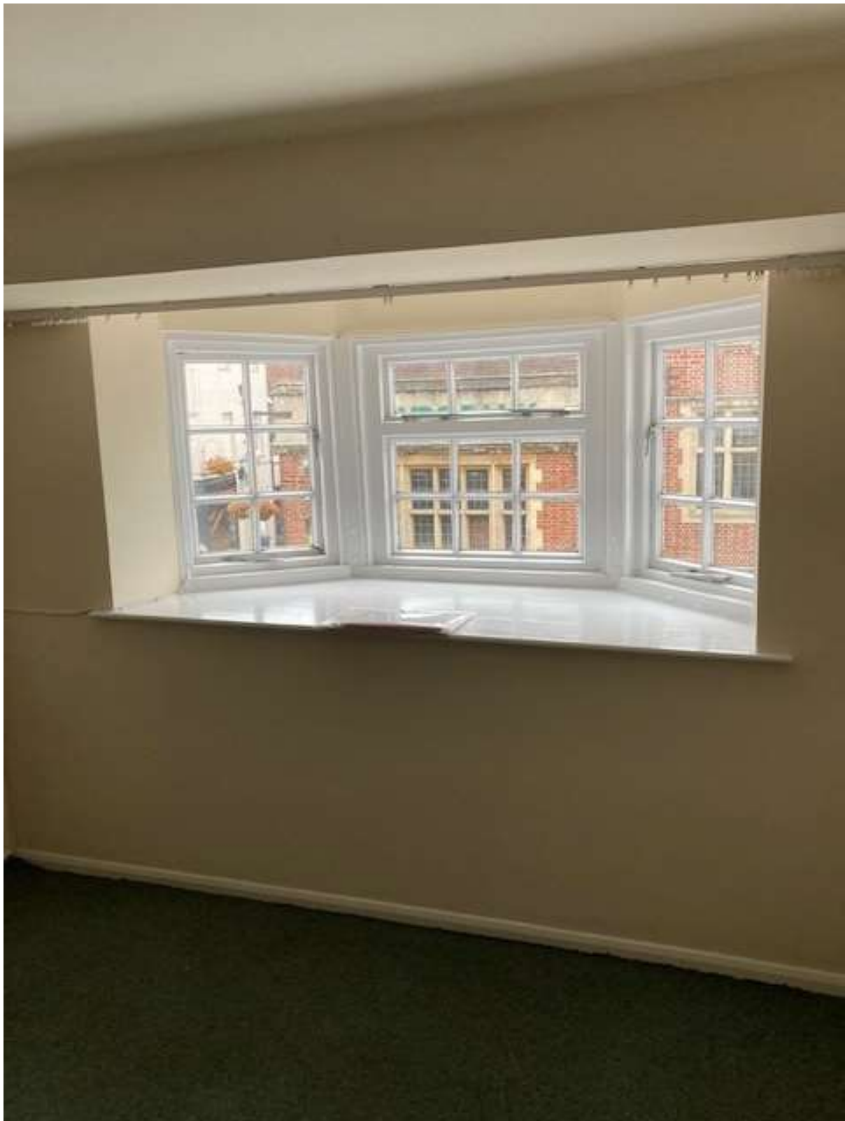
Figure 8: Canted bay window to living room (west elevation)
