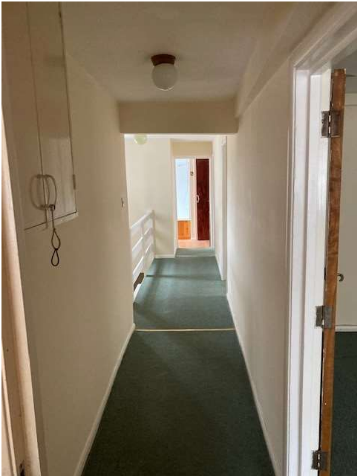
Figure 7: Stair hall and partition (part) for removal (from present kitchen door)
