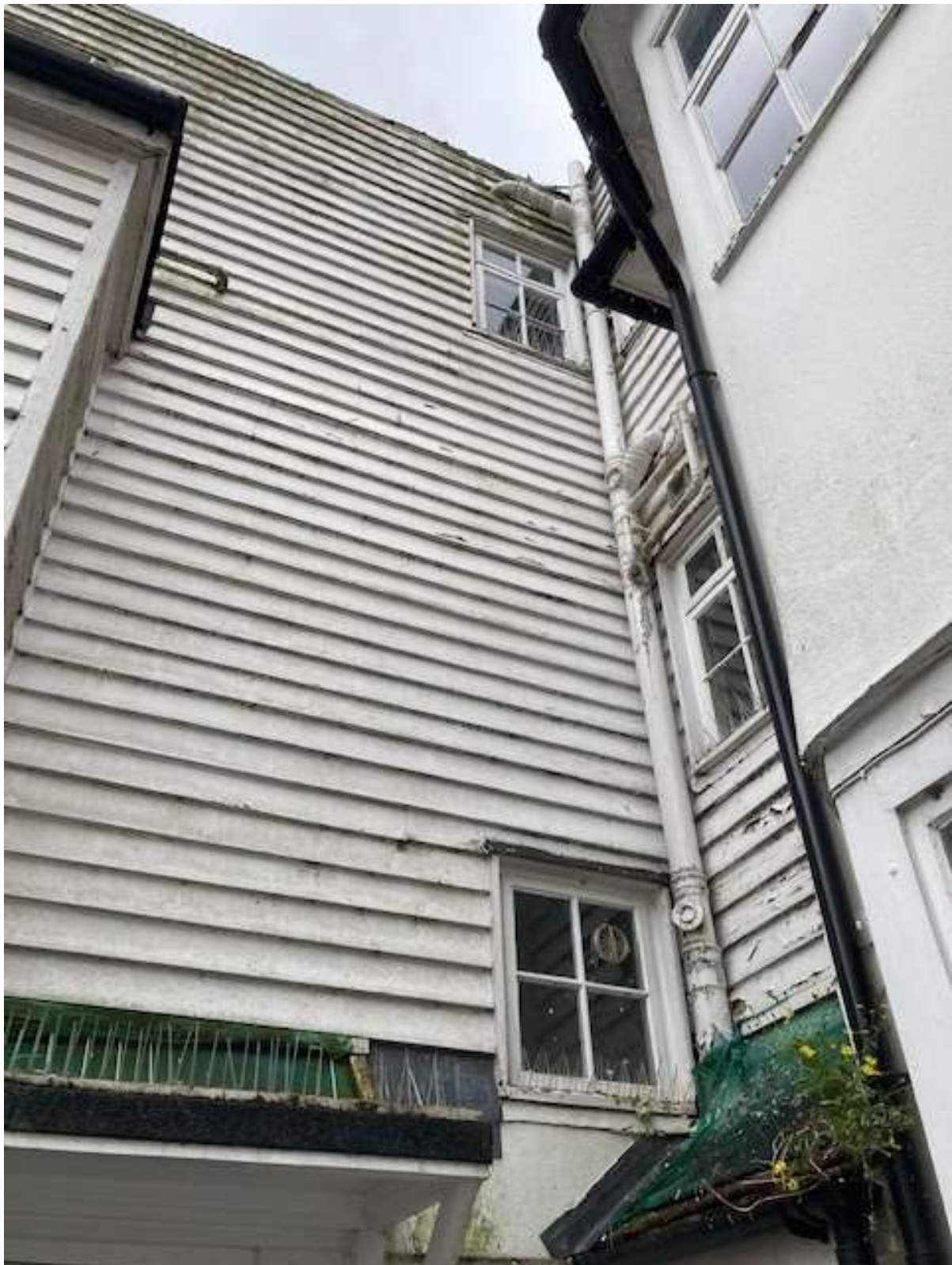
Figure 5: North elevation (adjacent to No.92)
