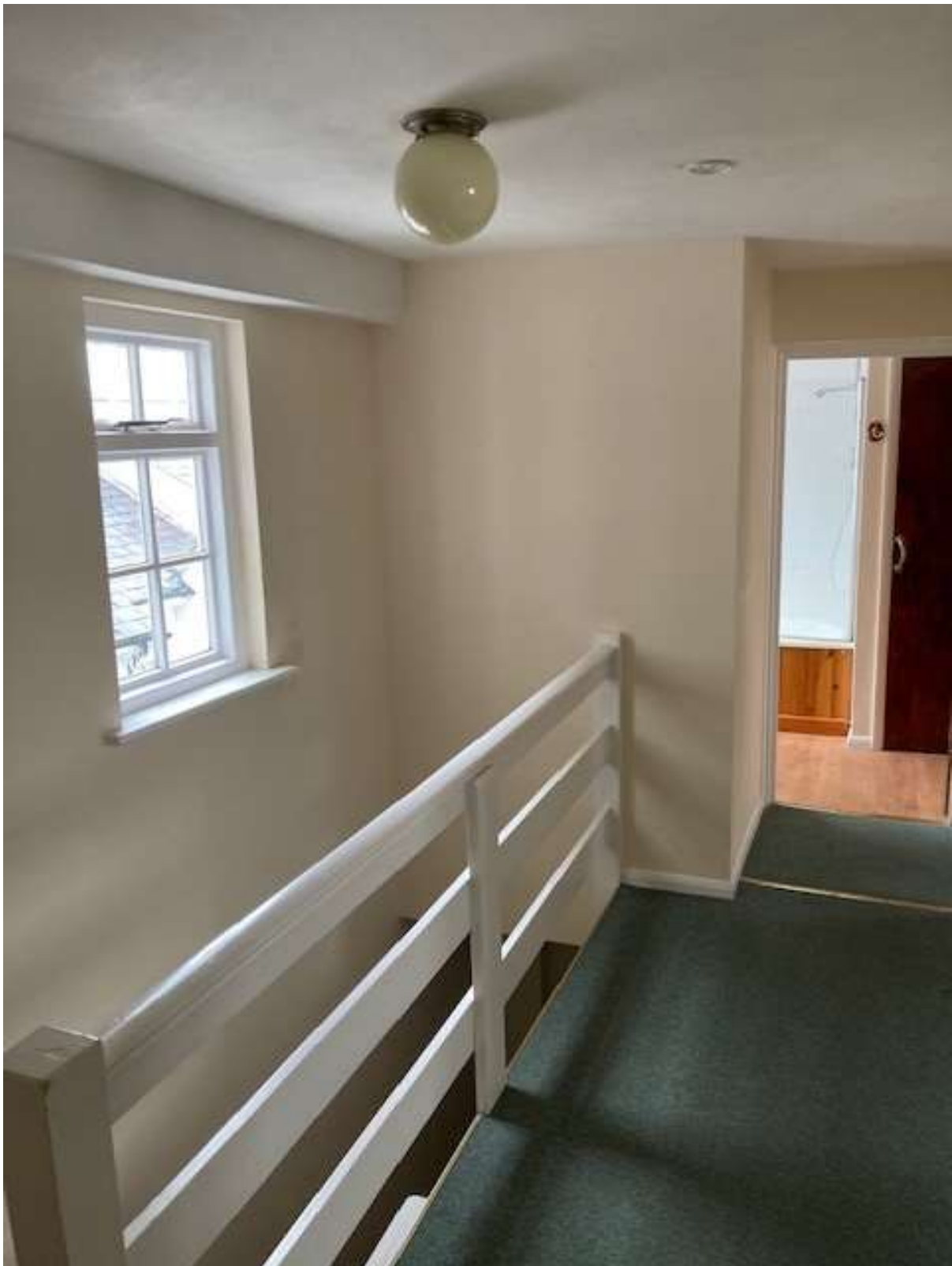
Figure 6: Flat 3: Stair and stair compartment/hall
