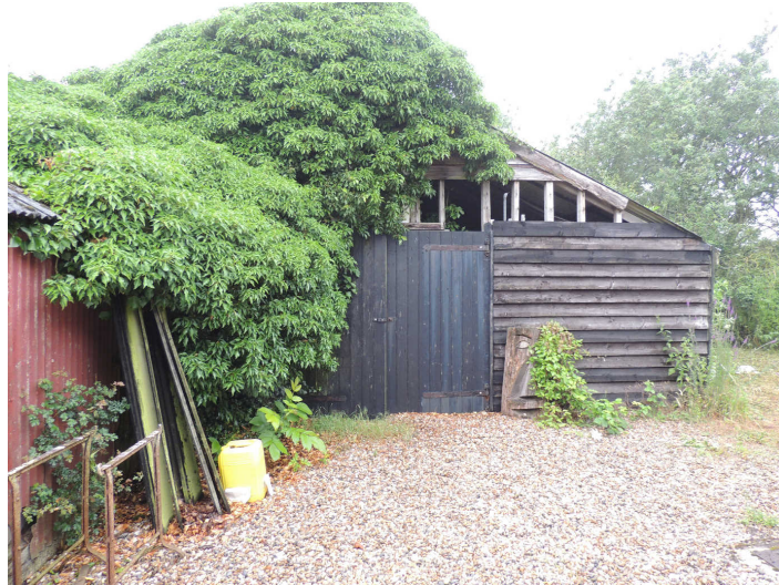
Photo 6: The eastern elevation is obscured by Ivy
