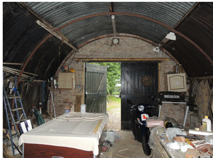
Photo 8: Looking eastwards in nissen hut
