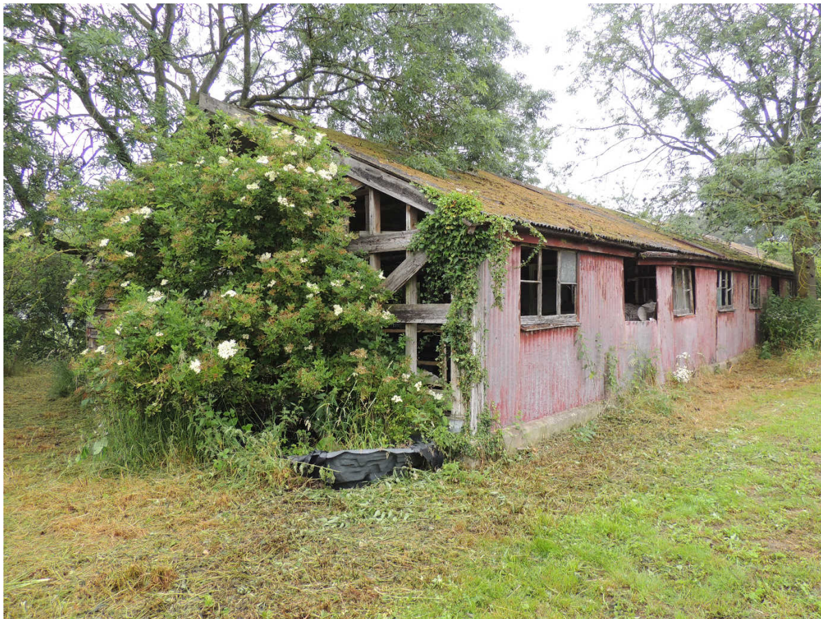
Photo 1: Western (gabled) and southern elevations
