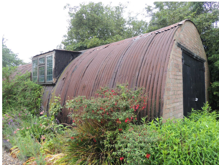
Photo 7: Eastern (end) and southern elevations of nissen hut
