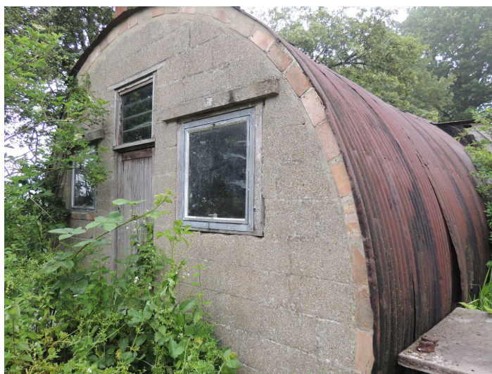
Photo 10: Western elevation of nissen hut
