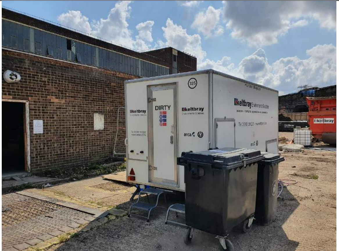
PLATE 9 Decontamination unit used during asbestos removal in the electricity substation within the D&E area.
