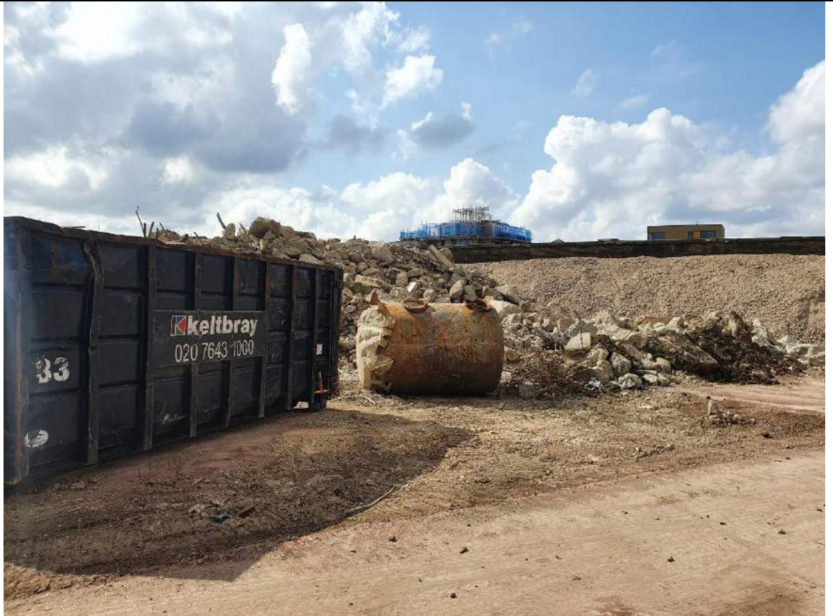
PLATE 4 One of the two buried tanks, this example was filled with concrete.
