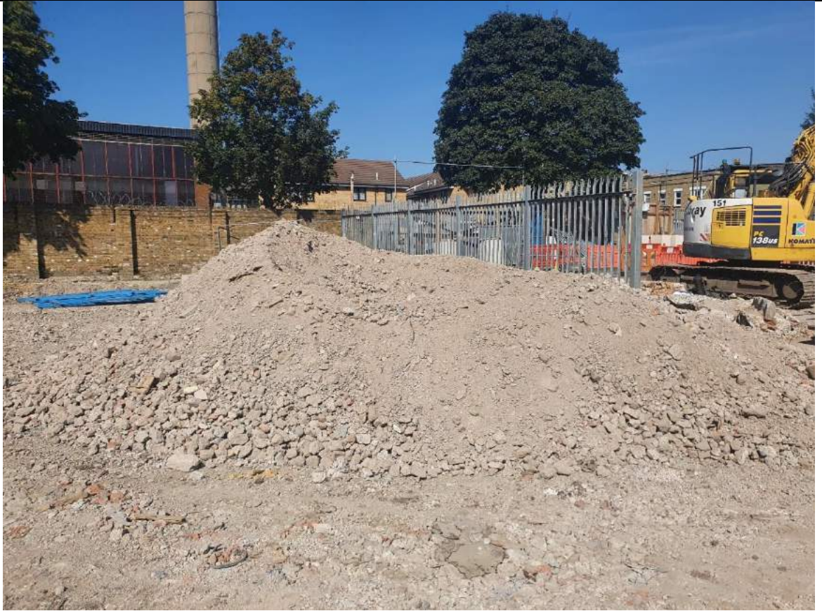
PLATE 10 Former electricity substation, now capped with crush.
