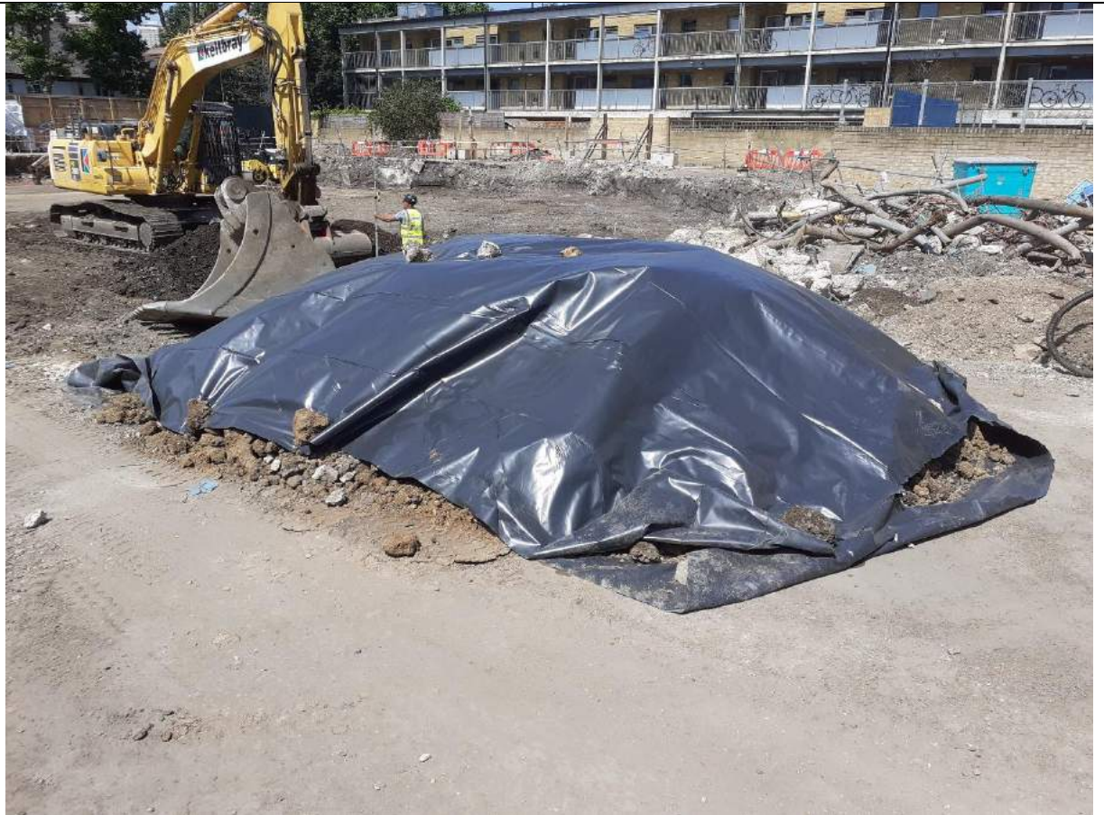
Stockpile of asbestos hot spot material, to be disposed of on Monday (26 th ).
