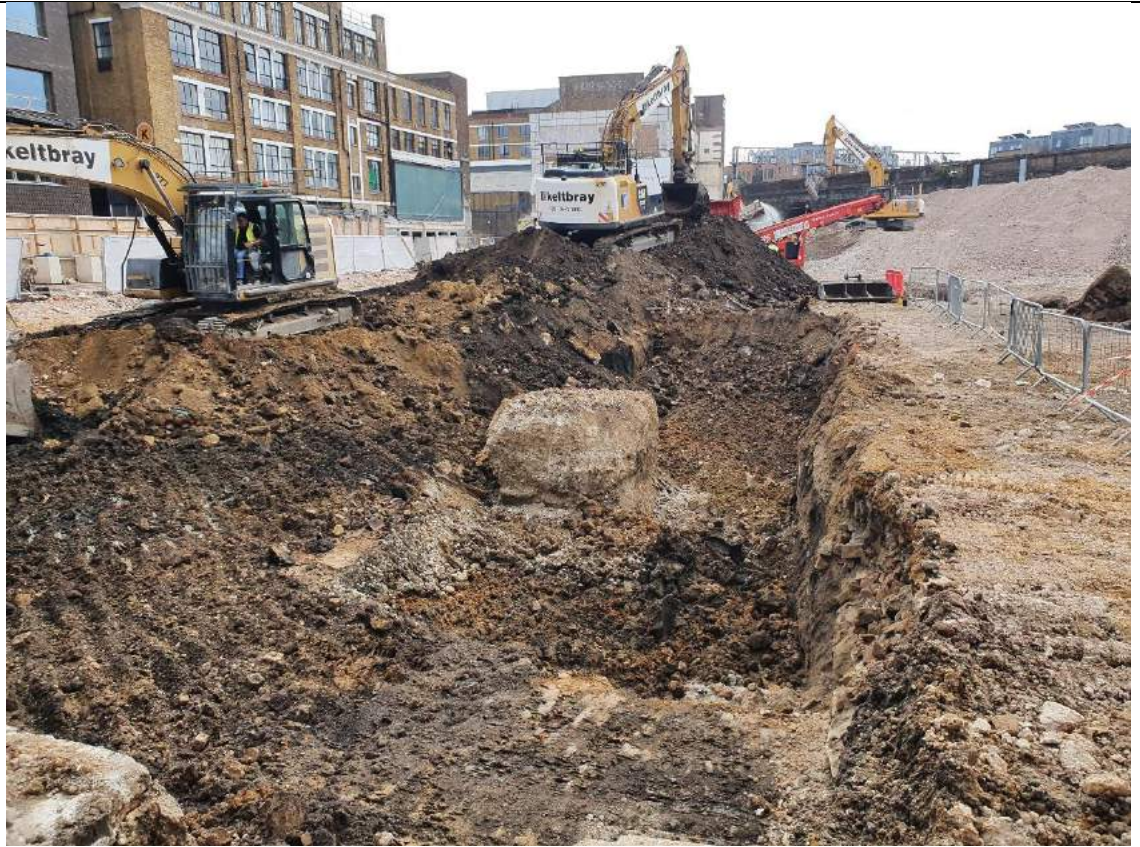
PLATE 7 Initial RST area excavations note the buried concrete.
