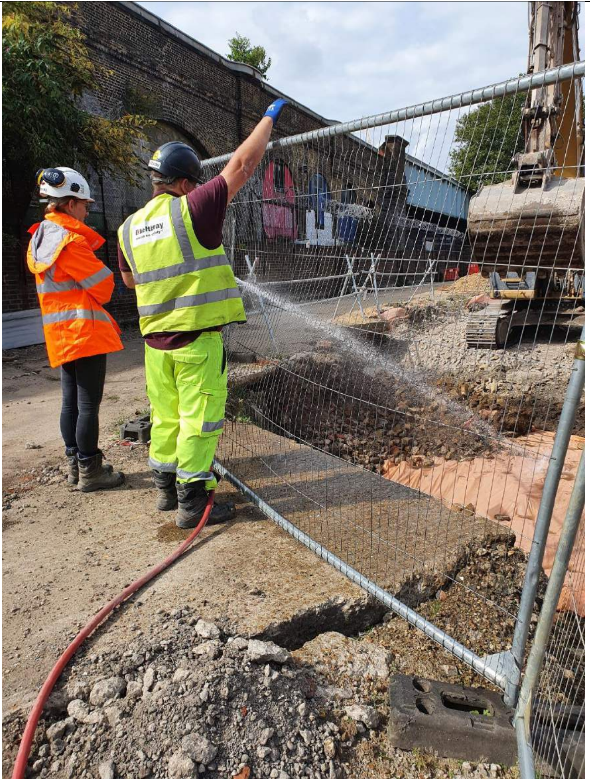
View looking north and down into the pit where the asbestos is being excavated. Also note the black soils at the base of said pit.
