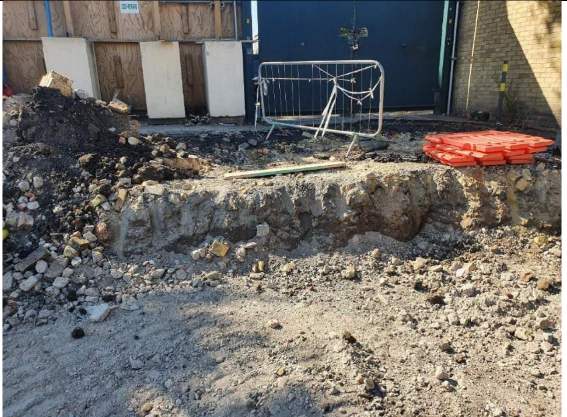
Soils to be cut back and then capped in the NW corner of Campus Site.
