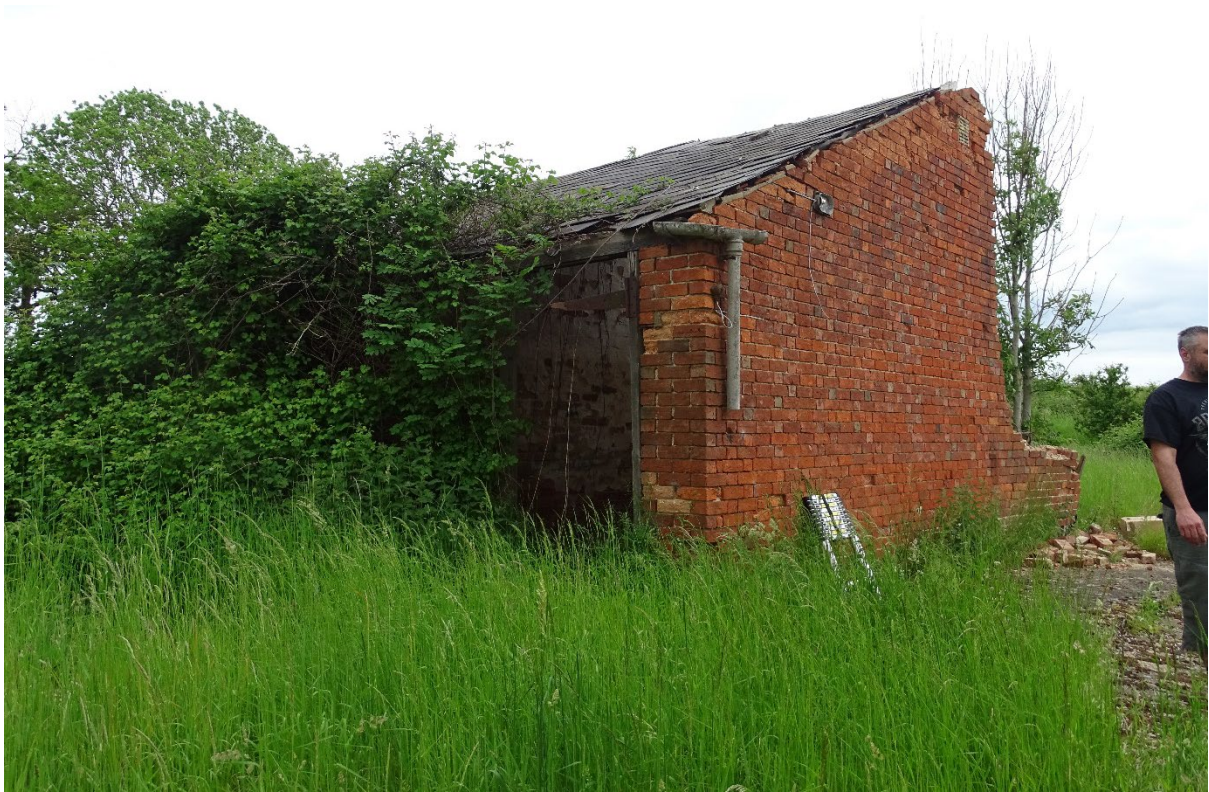
Image 14 – Building two, North & West facing elevation of the structure
