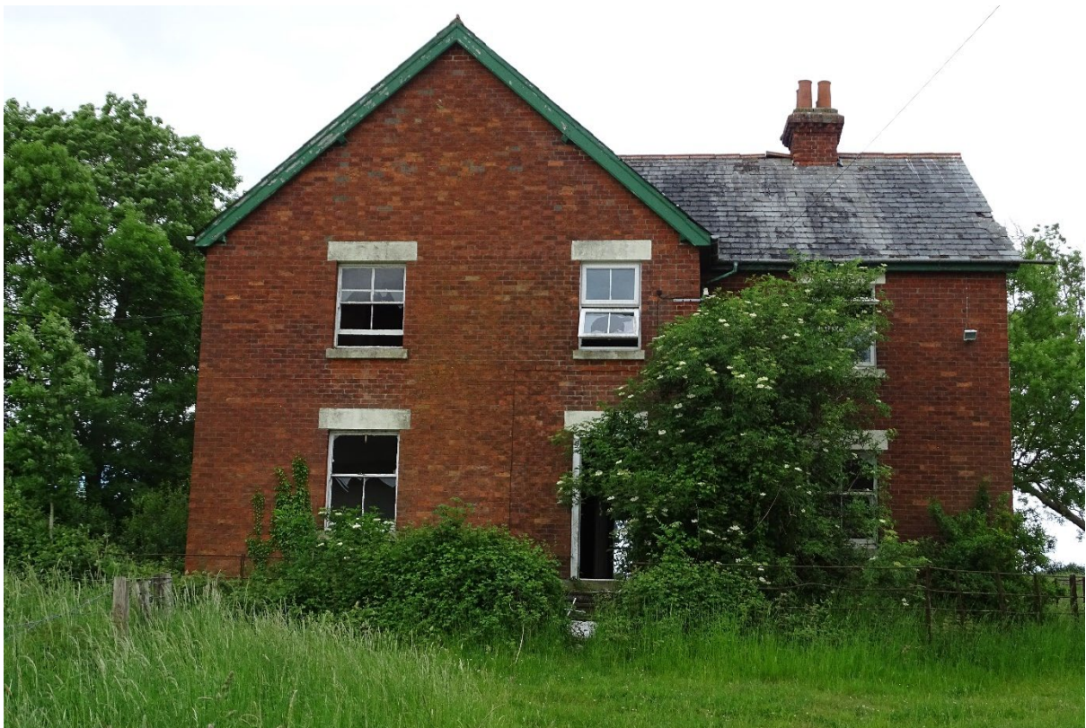
Image 9 – Building one – East facing elevation
