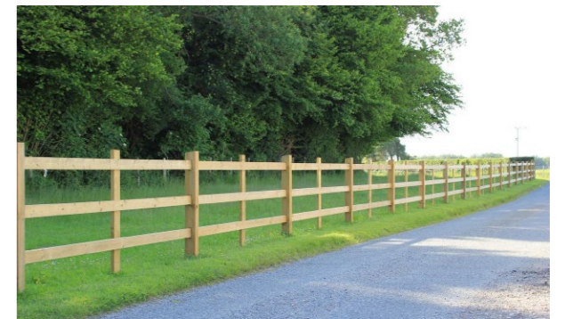
New 1.2m post and rail fencing to demarcate curtilage
