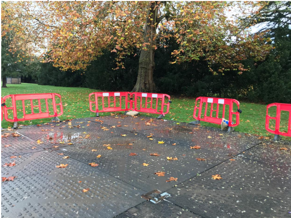
Photo 2. An example of heavy duty ground protection.
