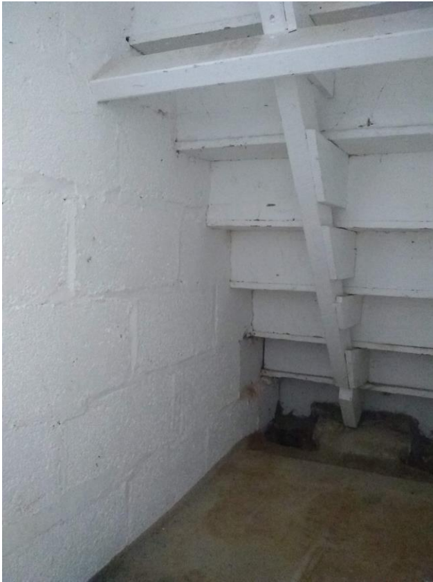
Figure 23: Later staircase from underneath. Adjacent is a later block wall, which is likely aligned with the location of an original wall
