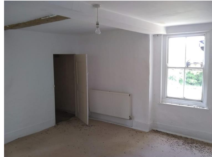
Figure 18: First floor bedroom within the later extension section. There is a downstand delineating the original gable wall. With the addition of the staircase and the extension, this room's planform is of no significance.
