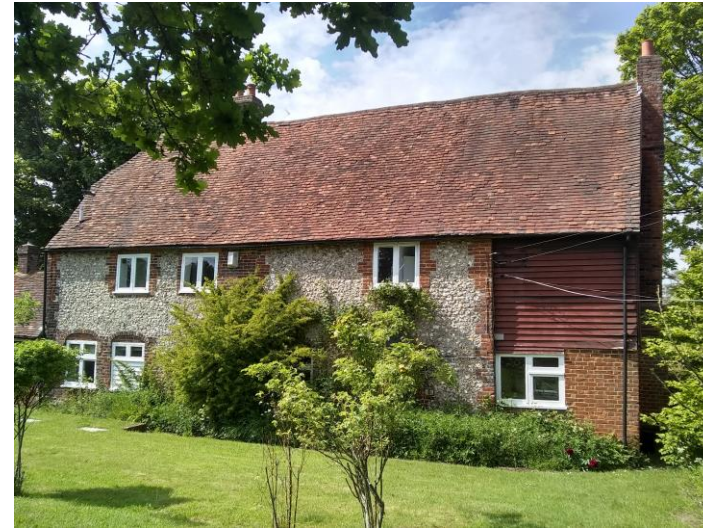
Figure 10: Rear elevation showing the later 20 th century two storey extension to the east gable wall
