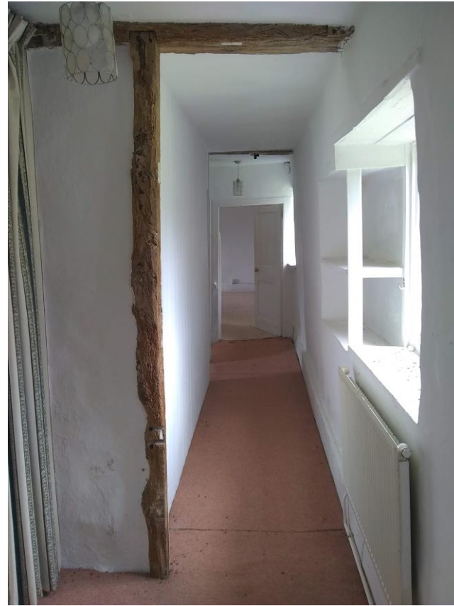
Figure 22: Hallway at first floor level. To the right hand side is the niche where there was a window originally.
