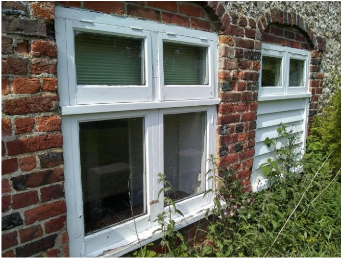
Figure 11: Later timber casement replacements which appear to be post 1950s
