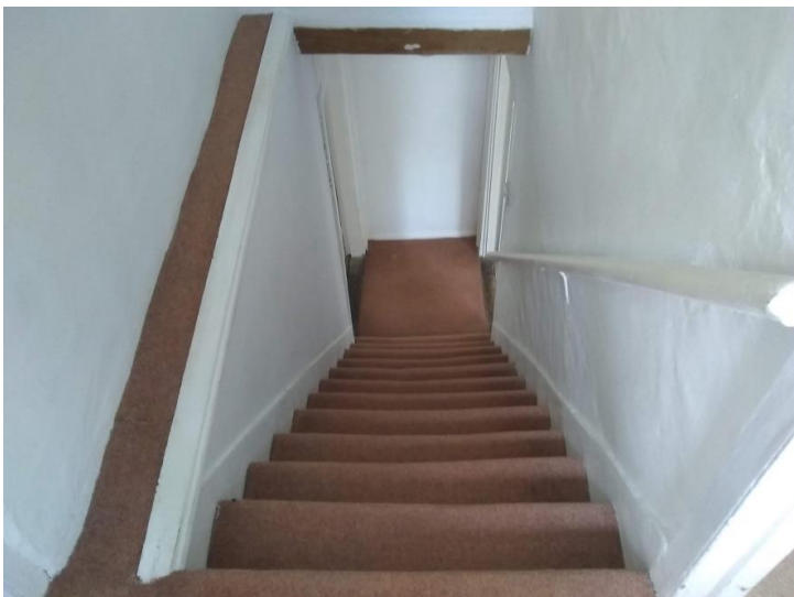
Figure 15: Later staircase likely added contemporaneously with the two storey extension
