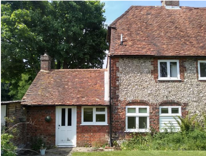
Figure 9: Rear elevation showing the hipped roof and the single storey extension
