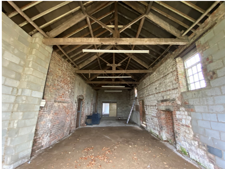
Plate 7 – stable, internal roof structure
