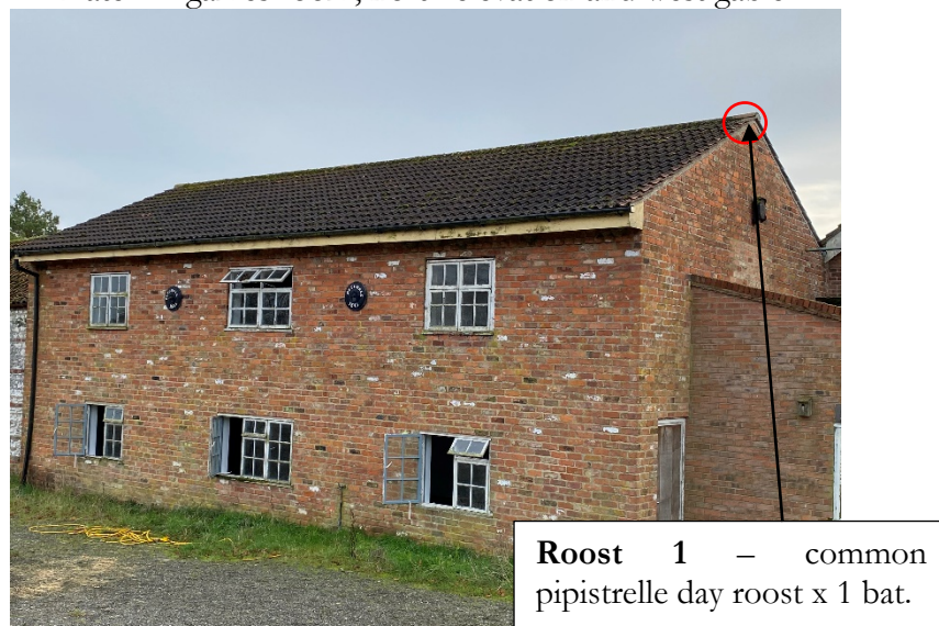
Plate 1 – games room, north elevation and west gable.
