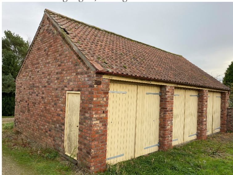
Plate 11 – garage 2, north gable and east elevation.
