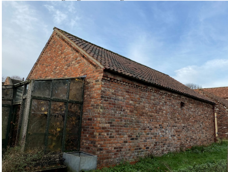
Plate 12 – garage 2, south gable and east elevation.
