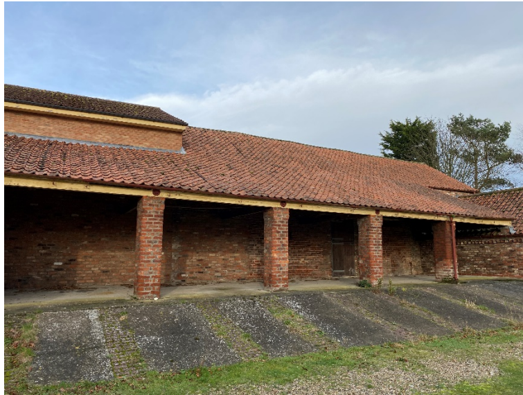
Plate 6 – stable, south elevation.
