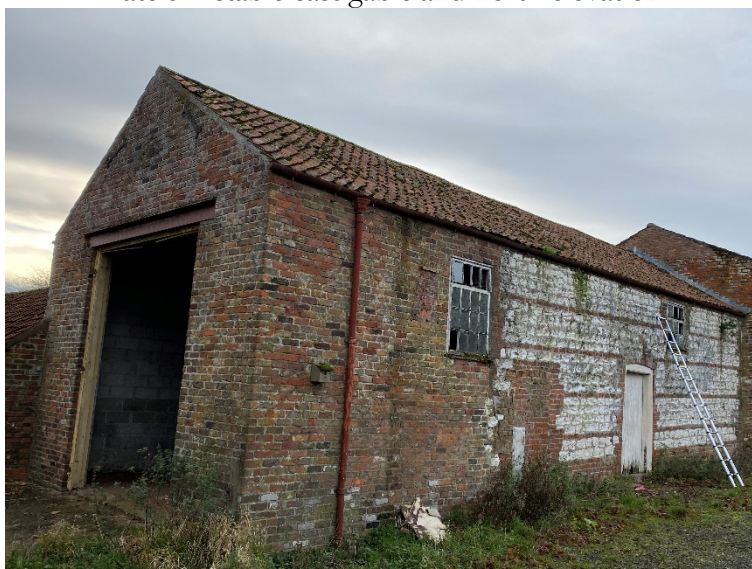
Plate 5 – stable east gable and north elevation.
