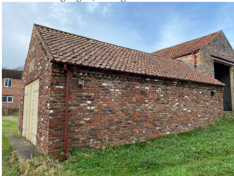
Plate 8 – garage 1, south gable and east elevation.
