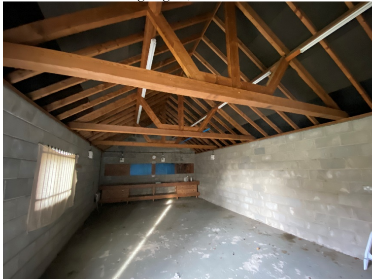
Plate 10 – garage 1, internal roof void.
