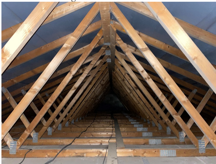
Plate 3 – games room internal roof void.
