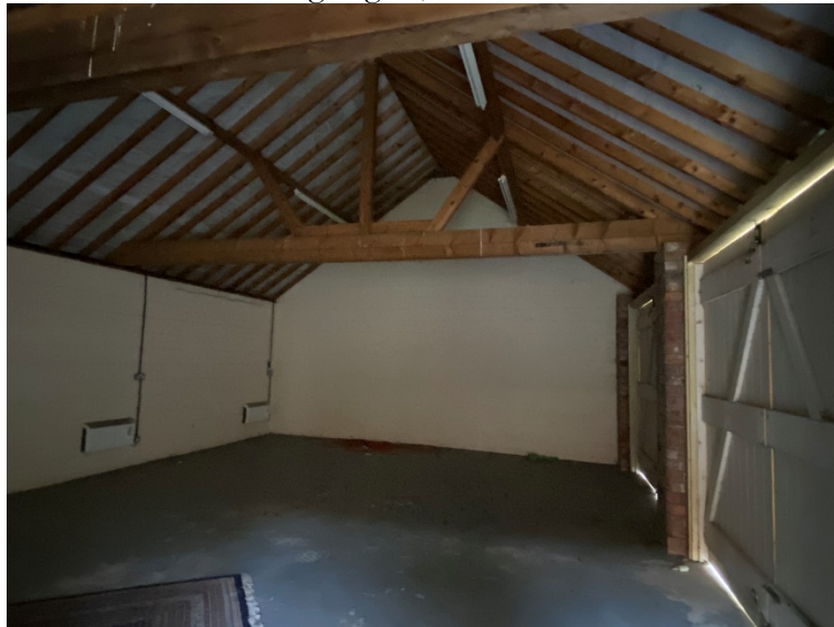
Plate 13 – garage 2, internal roof void.
