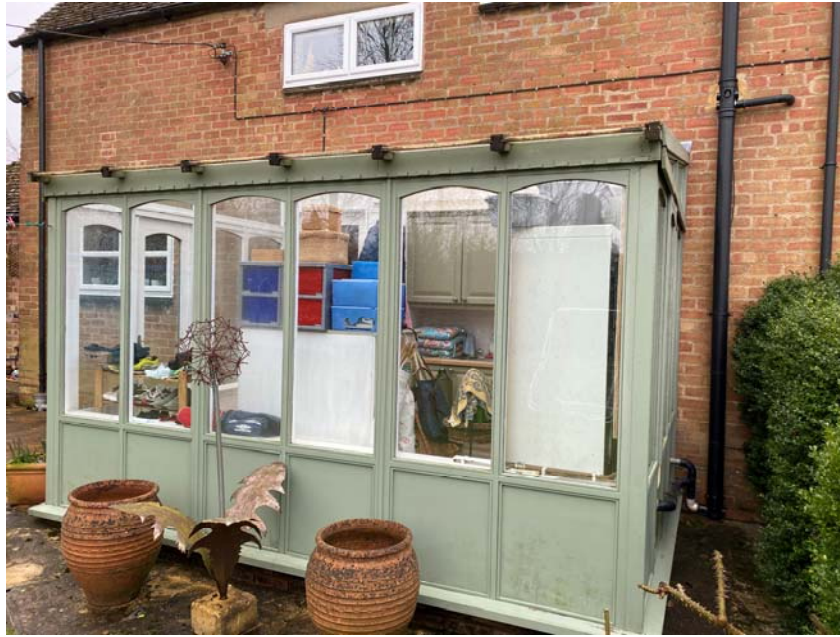
Above: existing conservatory
