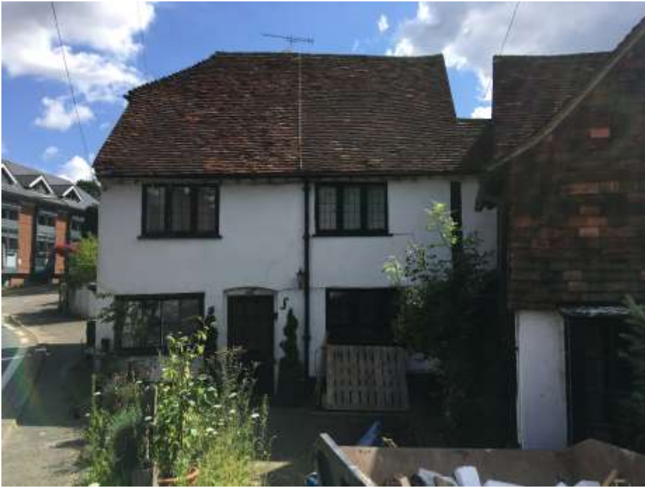
Photograph 4 Existing west elevation
