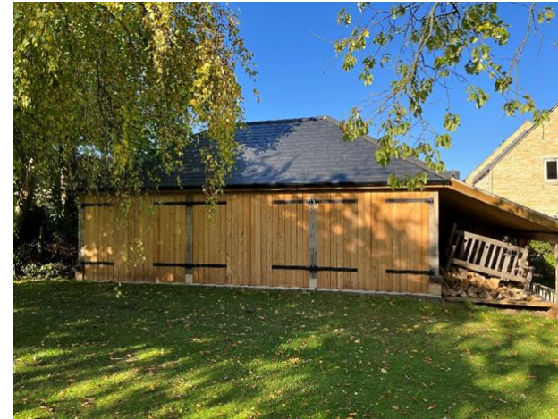
Figure 2: Oak frame garage – existing as erected
