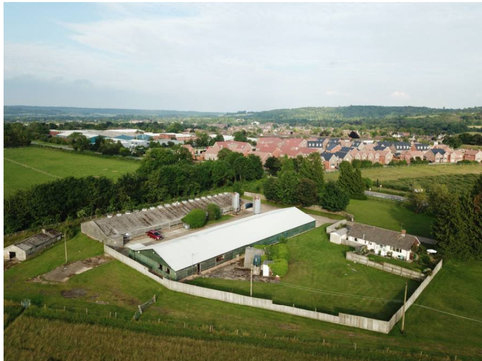
Image 8 – Existing Trees/Vegetation and Fencing Screening the Site
