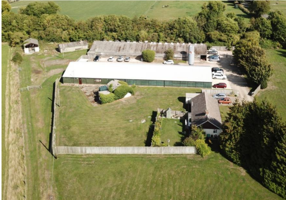
Image 5 – Existing buildings, fencing and planting on the Site
