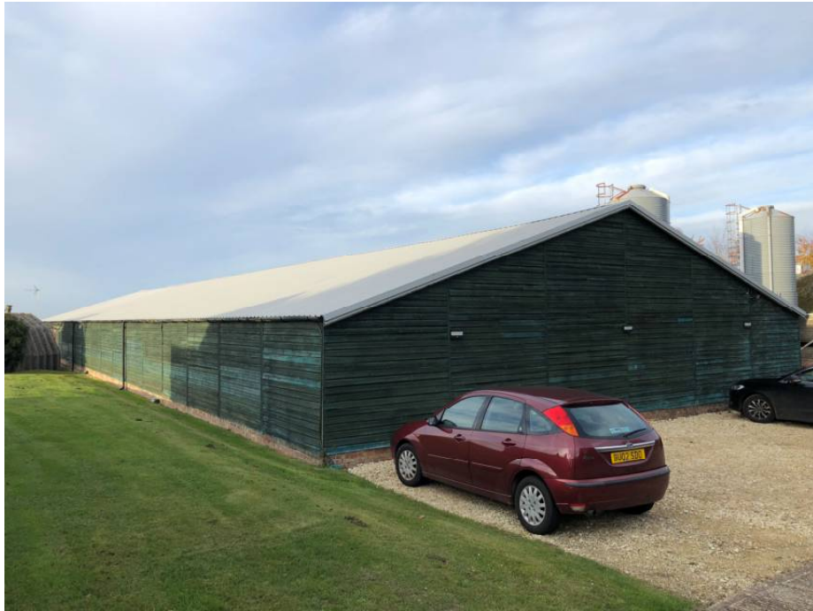
Image 3 – Existing Building & Silo – Shed A/Unit 1
