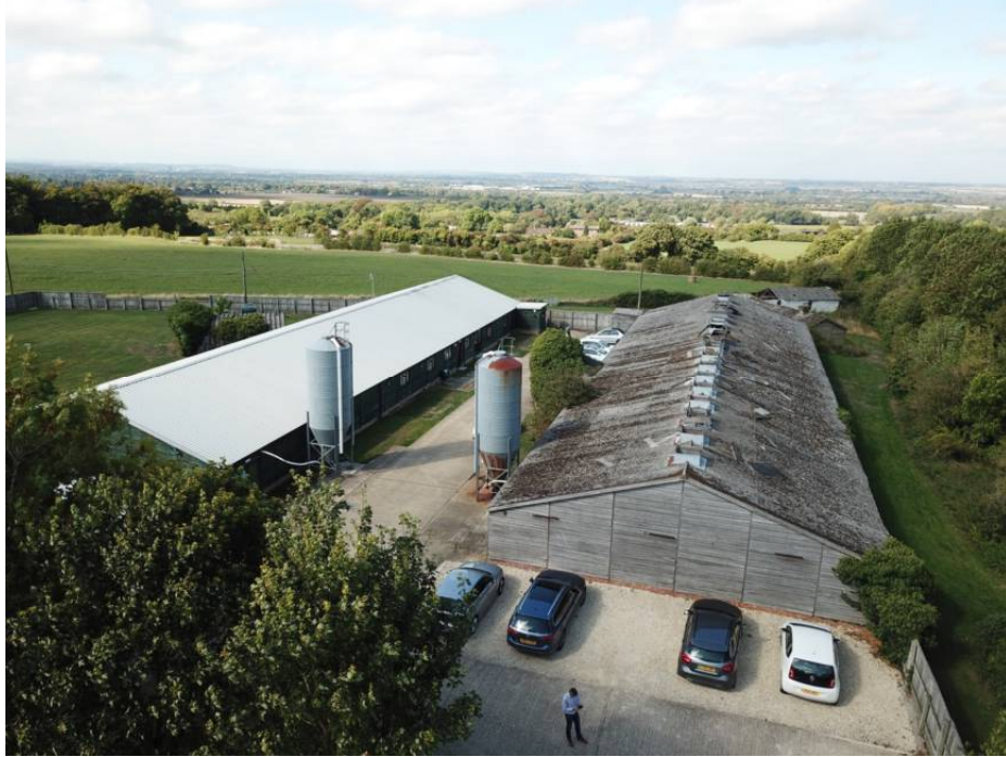
Image 4 – North-East Elevation of Shed A/Unit 1 and Shed B/Unit 2
