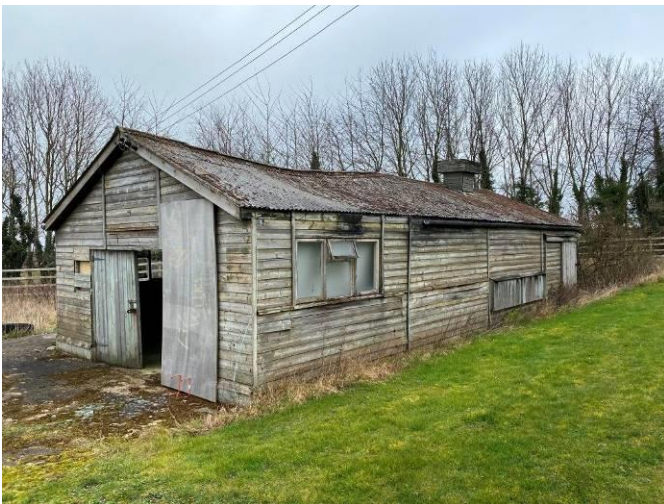
South and west elevations of Building 5
