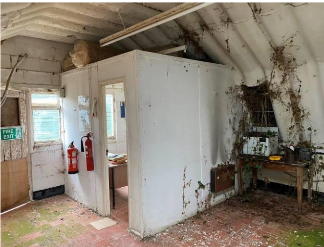
Enclosed office at north end of Building 3
