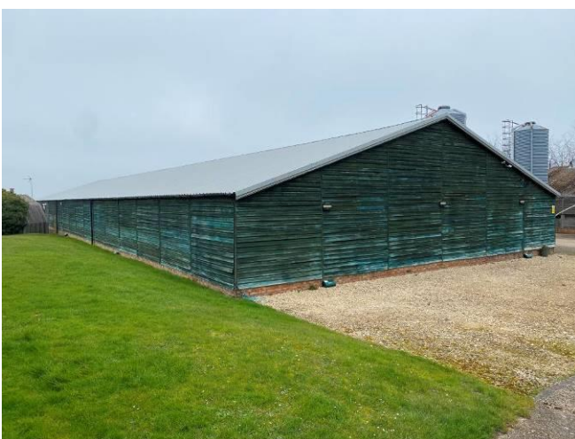
Southwest and southeast elevations of Building 2
