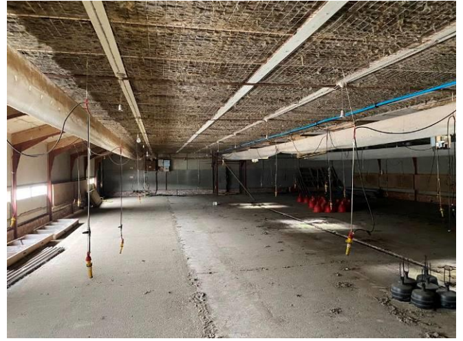
Interior of Building 1
