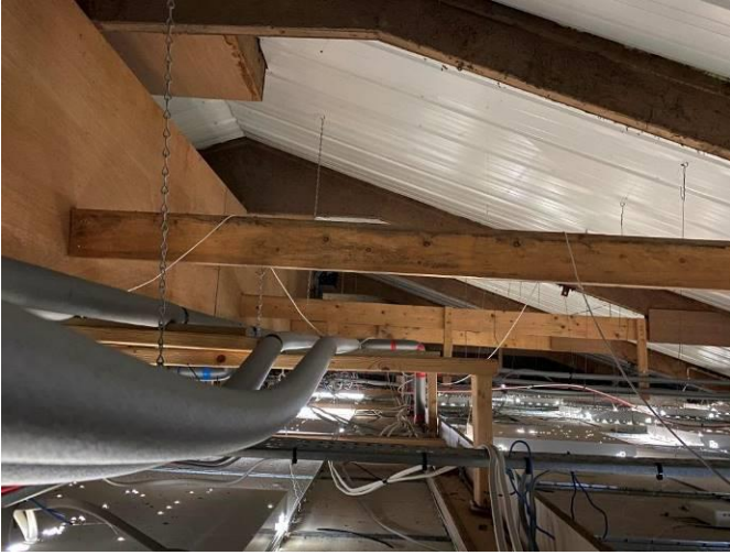
Roof space above offices in Building 2
