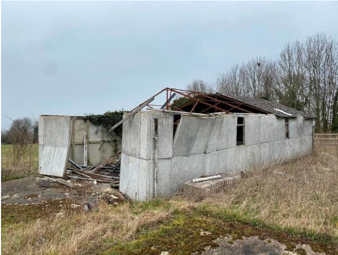
South and east elevations of Building 6
