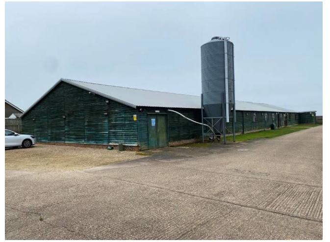
Southeast and northeast elevations of Building 2
