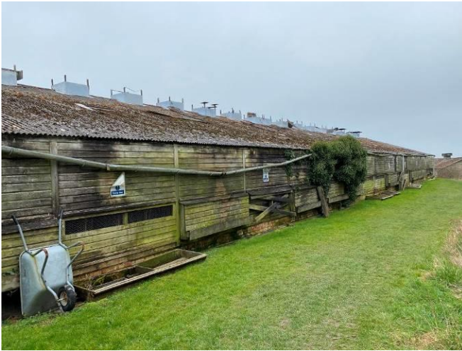
Northeast elevation of Building 1
