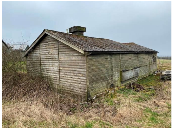
North and east elevations of Building 5
