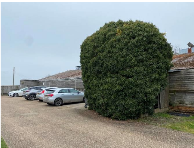
Side sections on southwest elevation of Building 1
