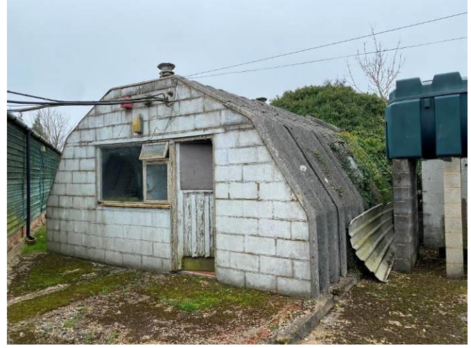
North and west elevations of Building 3
