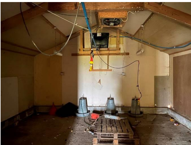
East room of Building 5
