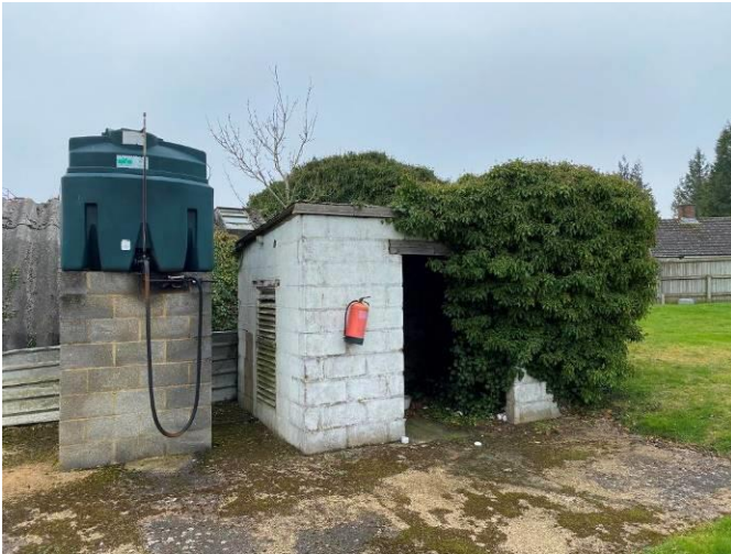
North and west elevations of Building 4
