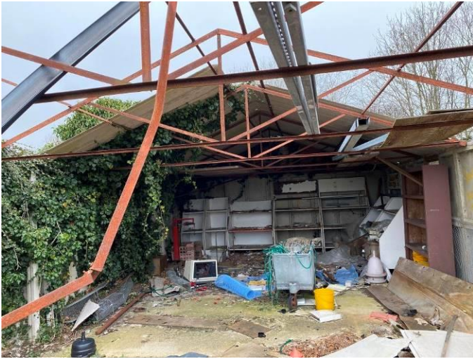
Interior of Building 6
