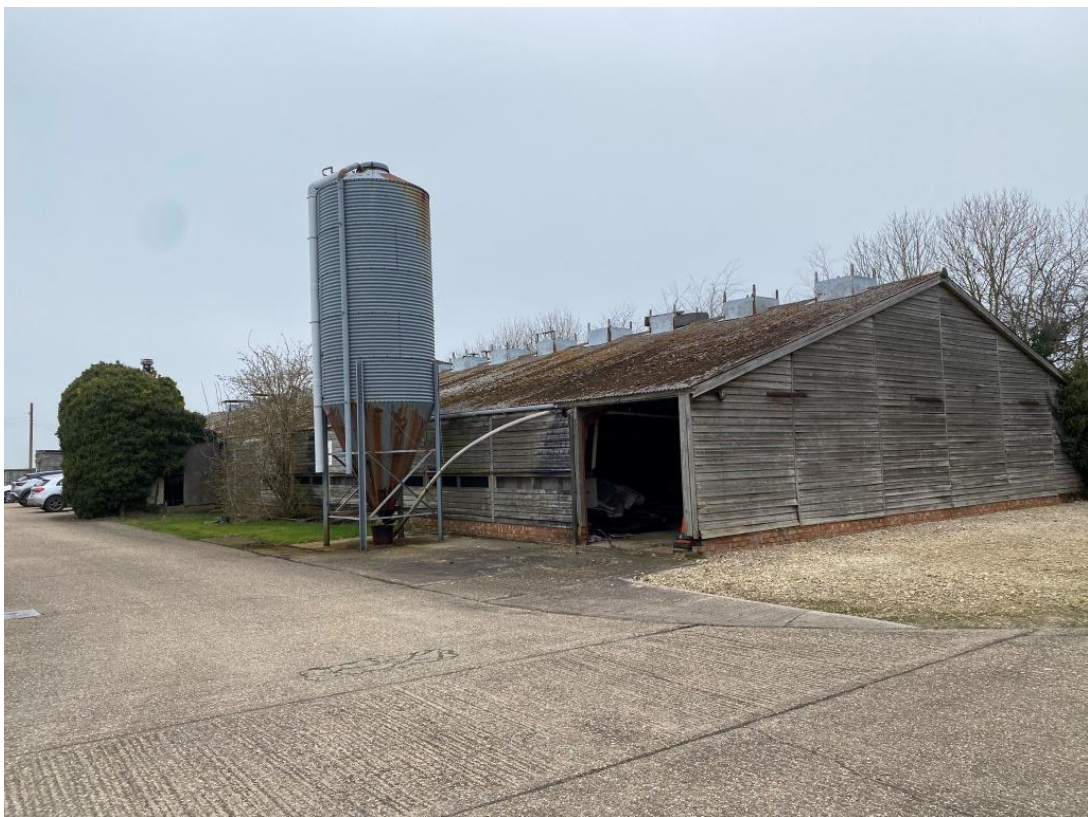
Southeast and southwest elevations of Building 1
