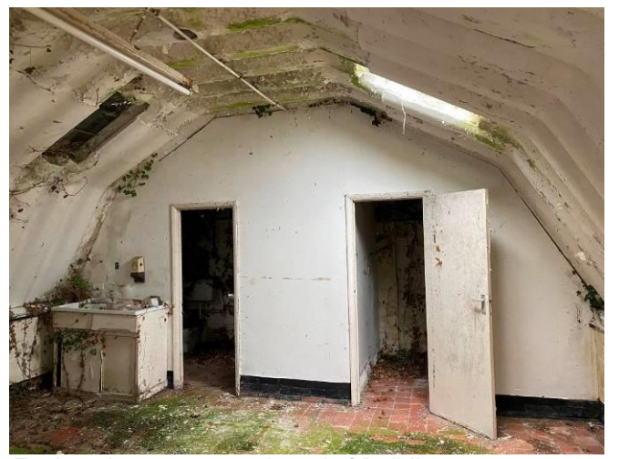
Enclosed rooms at south end of Building 3
