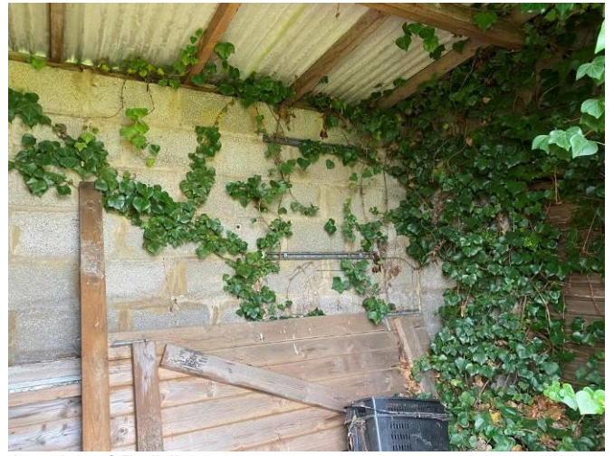
Interior of Building 4
