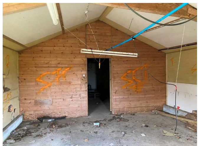
West room of Building 5
