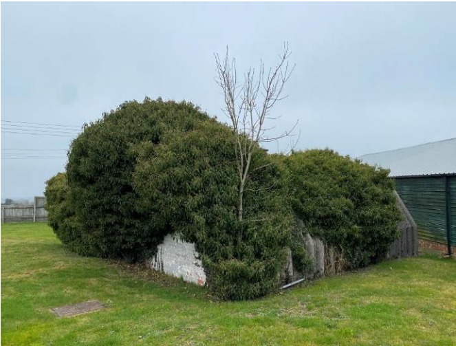
South and east elevations of Building 3
