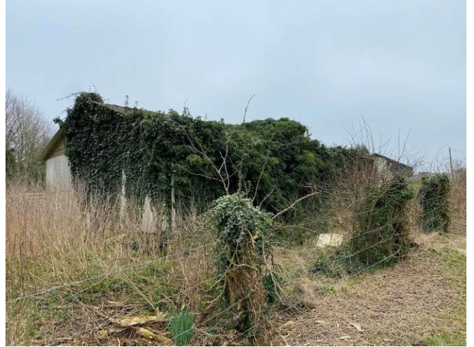
North and west elevations of Building 6
