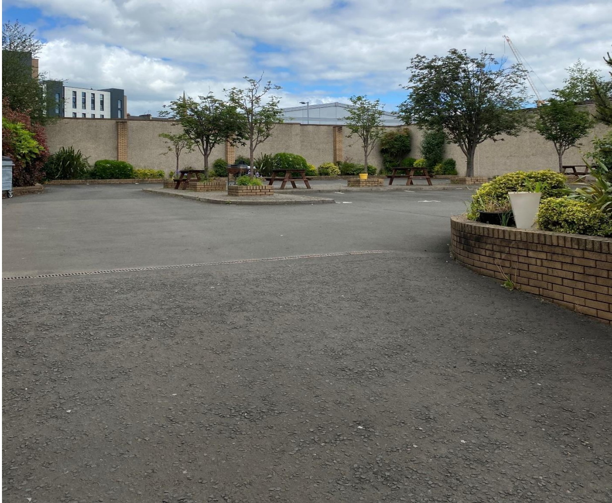
Plate 3 Rear Car Park
