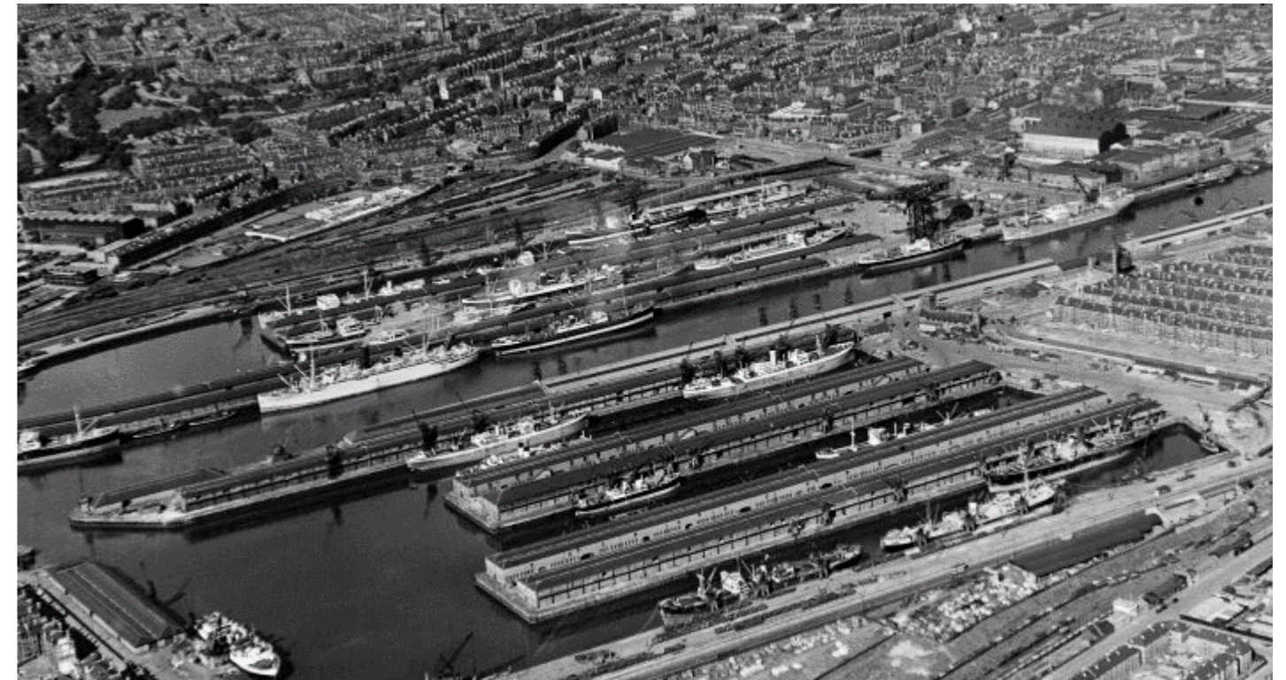
Figure 3.2 Late 20th century aerial photograph of Queens Dock. (Source: Canmore)
