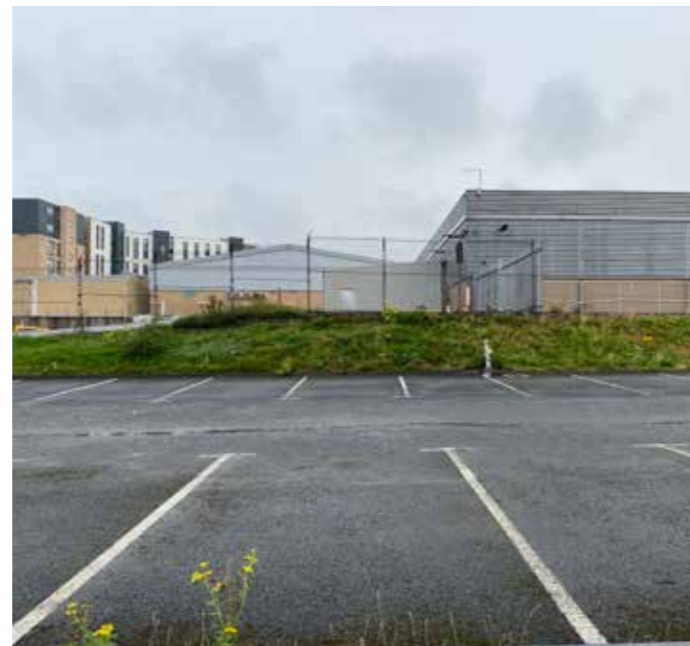
Figure 6.5 View from West Greenhill Place looking north across a car park to the rear of the business park development
