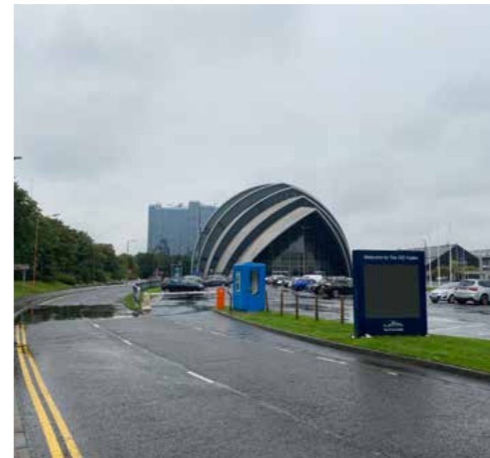
Figure 6.6 View looking east along Congress Way with the Crowne Plaza in the background
