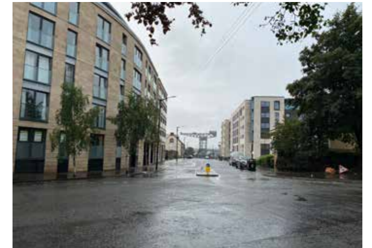
Figure 4.6 View looking south along Minerva Street
