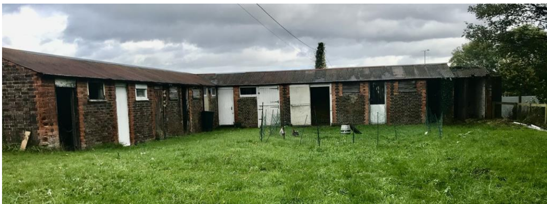
Fig 5: North and west elevations of huts looking east.
