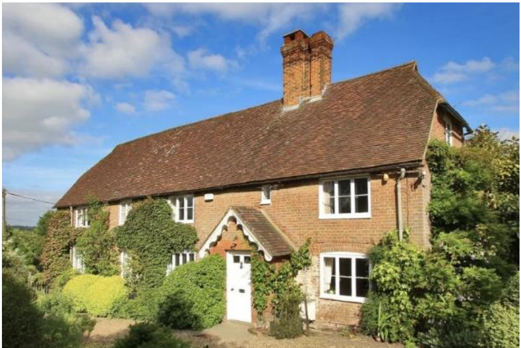
Fig.3: Northwest elevation of farmhouse.
