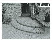
A low level brick wall retained the front garden adjacent the property which was noted to be structurally sound with no failure noted.
