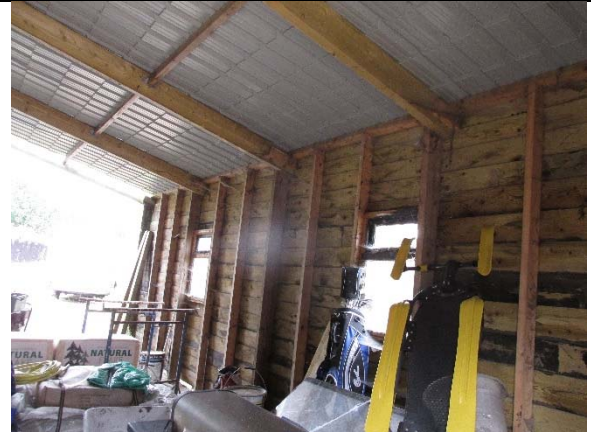
Plate 14: Interior of the lean-to of S1
