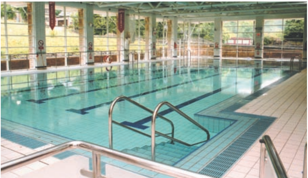
Todmorden Sports Centre – permanent ‘easygoing’ access incorporated into the pool
