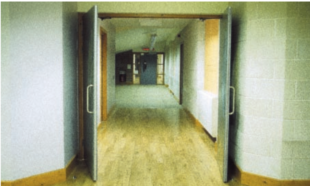
Whenever possible doors should be held open to minimise the number of barriers on a route way. Splayed walls at corridor junctions will benefit visually impaired people and wheelchair users
