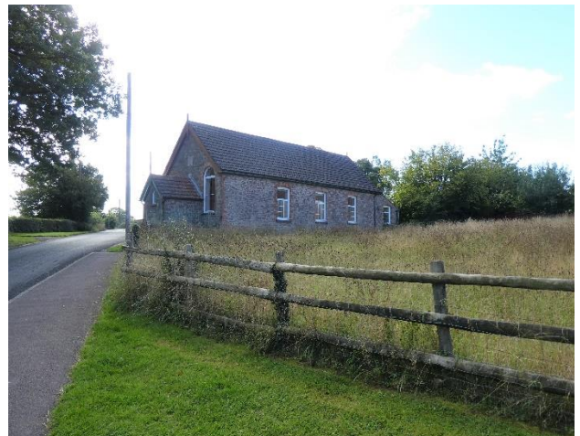
From north -west , over adjoining field.
