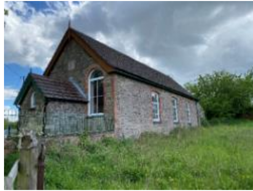
Plate 2: Western elevation and adjacent pasture field.
