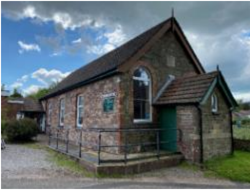
Plate 1: North-east elevation showing the original Church (section 1) and front porch (section 4).
