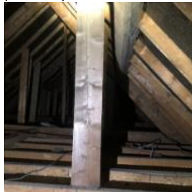
Plate 12: Square cut timbers in good condition in the loft void.
