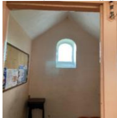
Plate 8: Interior of the porch (section 4).
