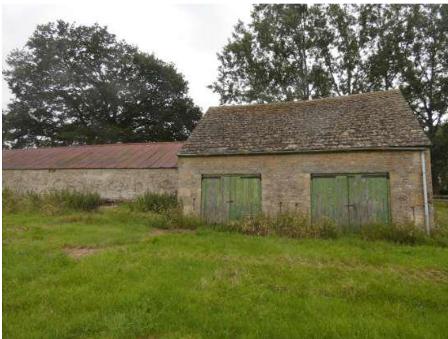
Figure 2:1: East elevation of existing barn
