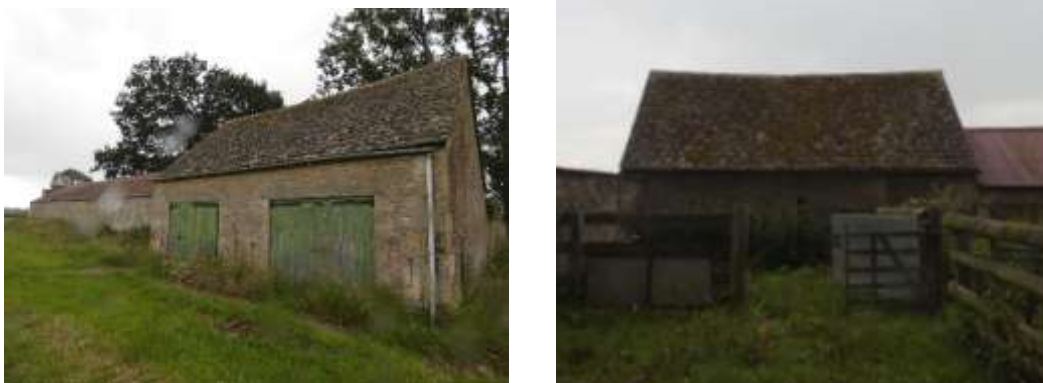
Figs. 5 & 6 Roof of stone barn
