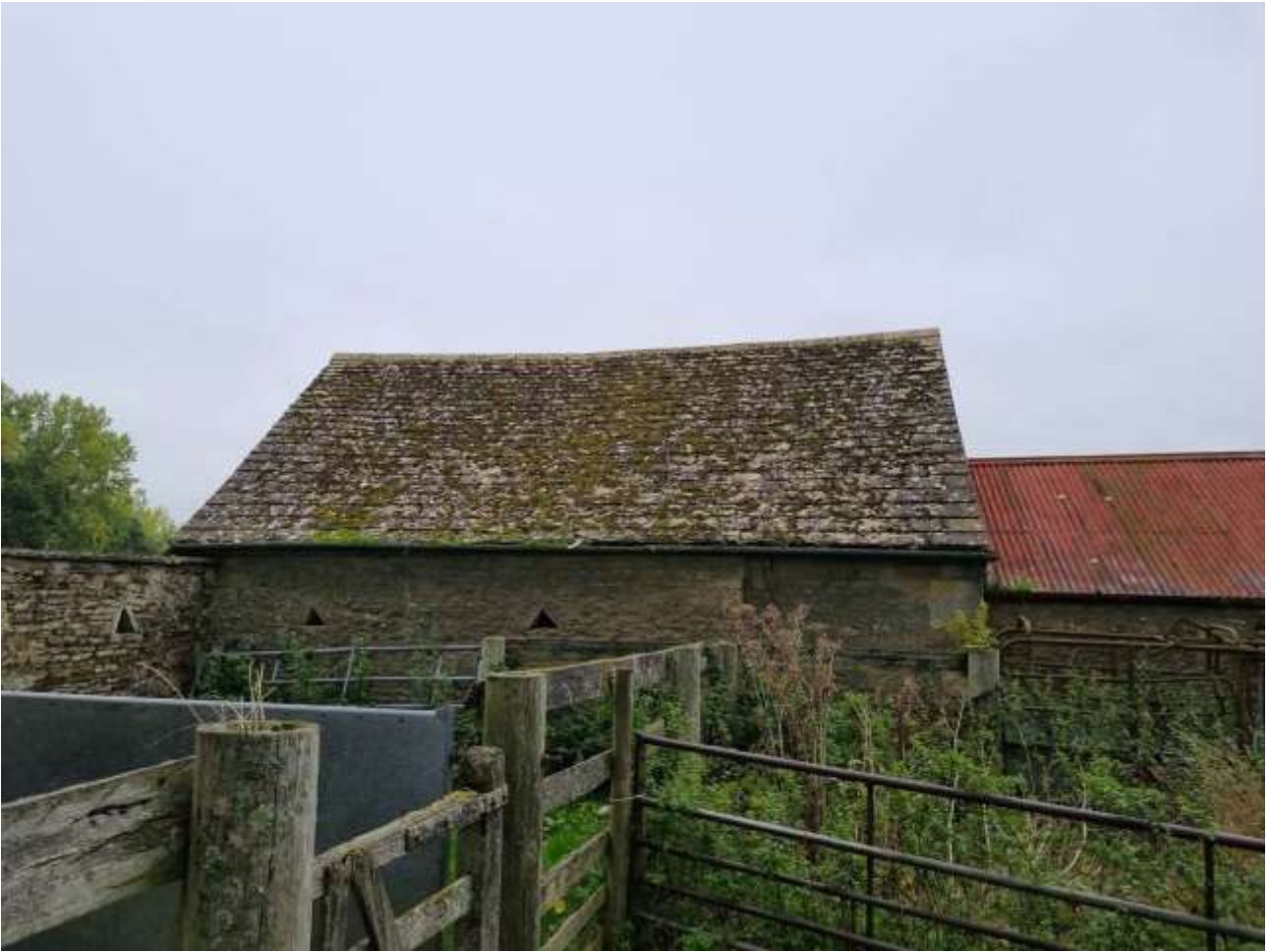
Photograph 3: Showing Western Elevation
