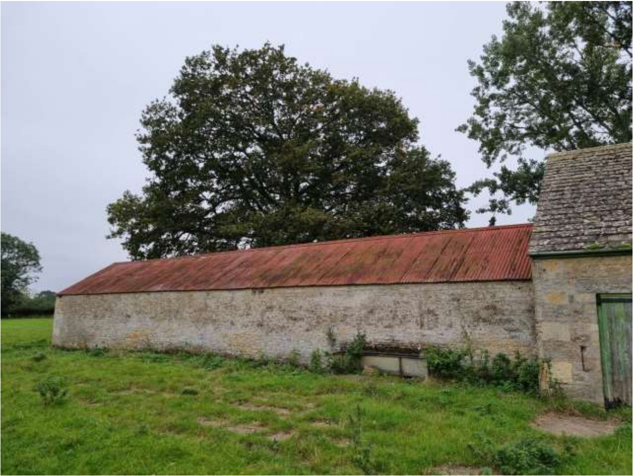
Photograph 2: Showing Eastern Elevation
