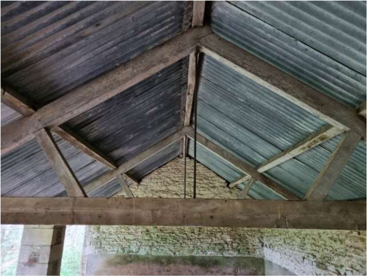
Photograph 5: Showing roof structure to Southern Part of Barn
