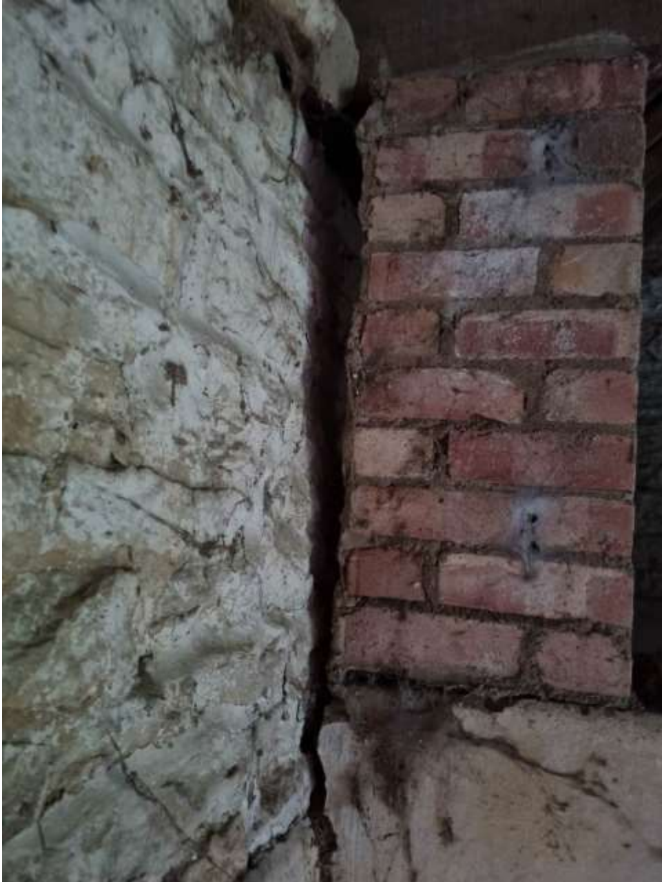
Photograph 7: Showing brickwork pier
