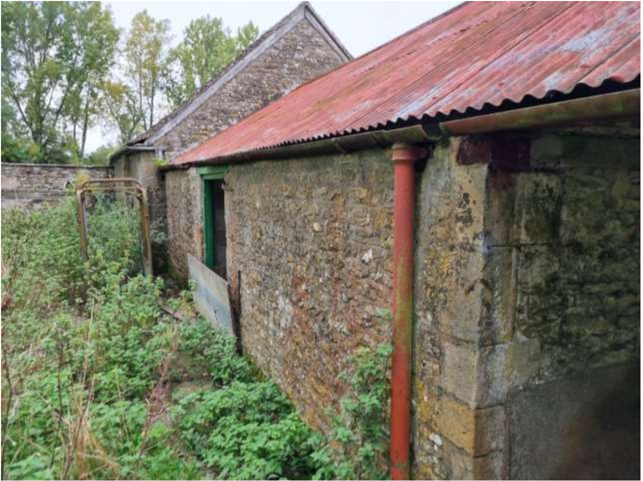
Photograph 4: Showing Western Elevation
