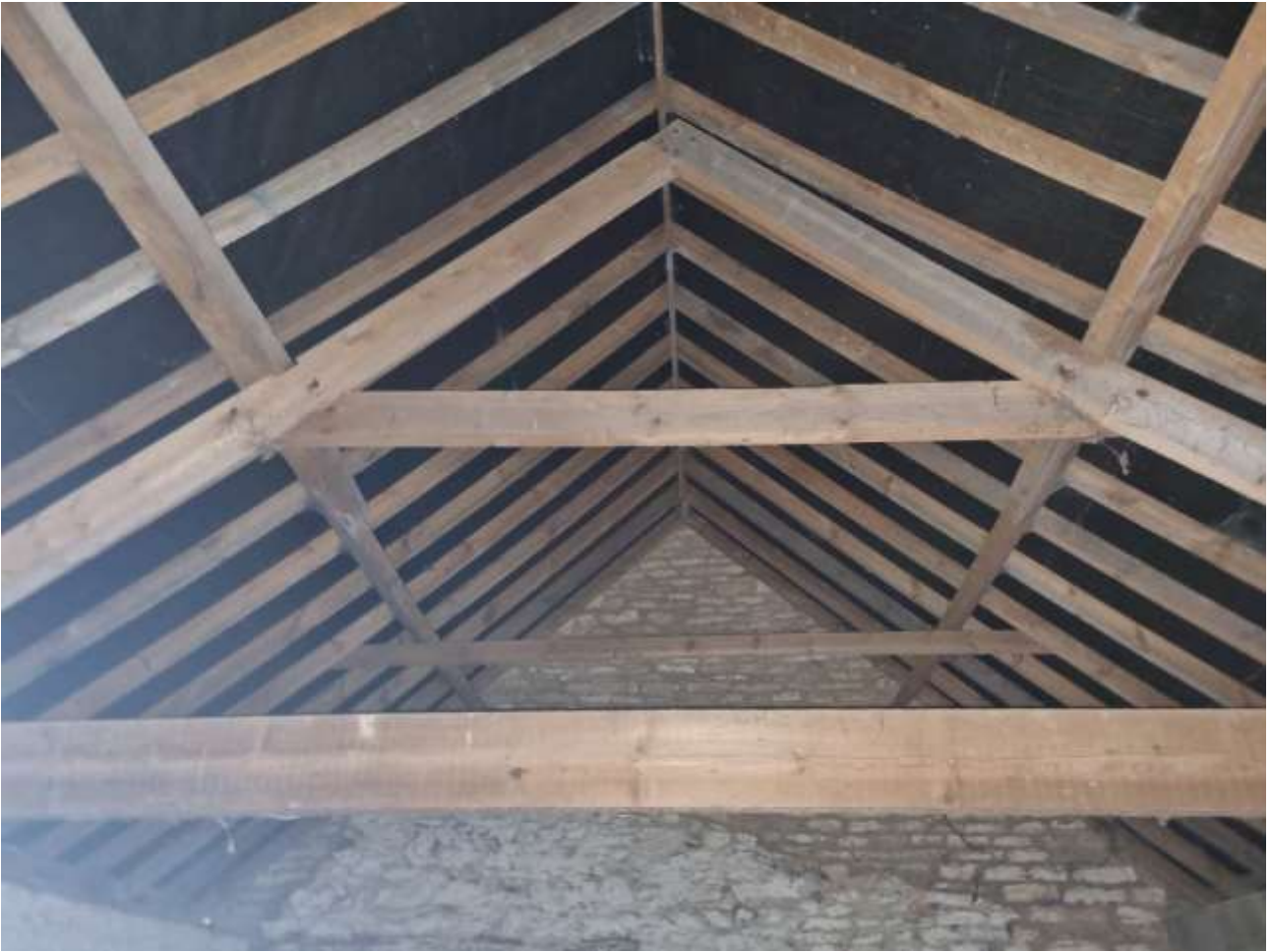
Photograph 8: Showing roof structure to Northern Part of Barn
