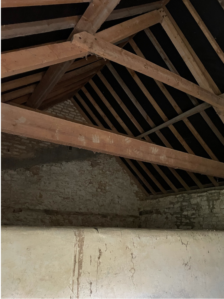
Fig. 5: Existing modern rod structure to main barn.
