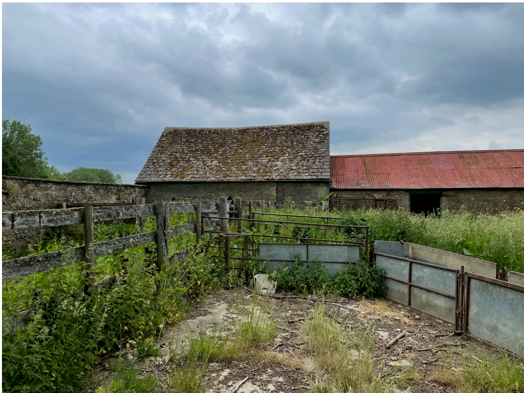
Fig. 2: Hard standing area where original barn extension stood.
