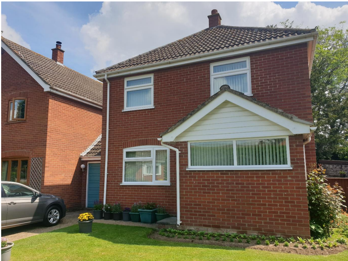
Figure 1: The front (West) elevation of the property, showing garage to the left and the single-storey porch to the right, which is to be replaced with a larger extension.
