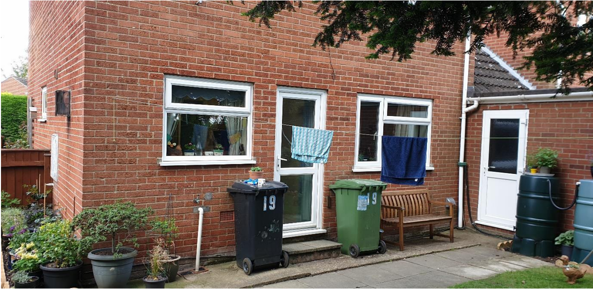
Figure 2: The rear (East) elevation of the property, showing the existing garage to the right. The new extension will start from the side wall on the left and run parallel to the house until it meets the garage wall on the right.
