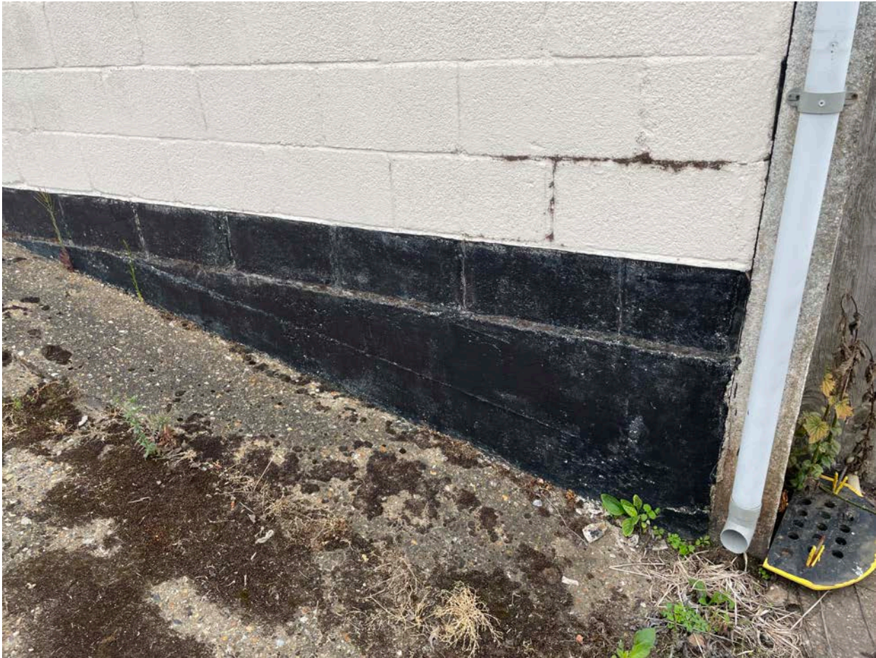
Image 6.0: Access ramp, local to opposite gable end with lower mass concrete set to underside of blockwork.
