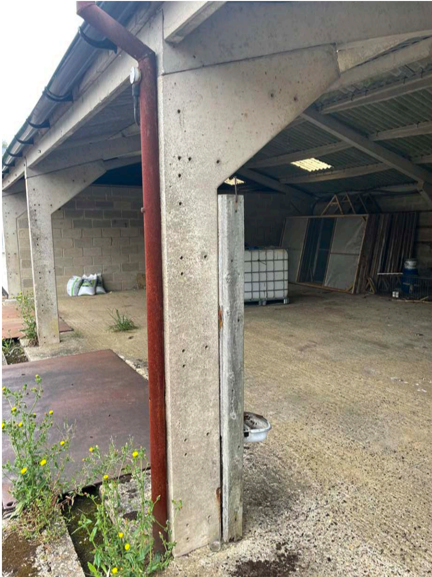
Image 5.0; View of concrete columns/ stanchions with haunches.
