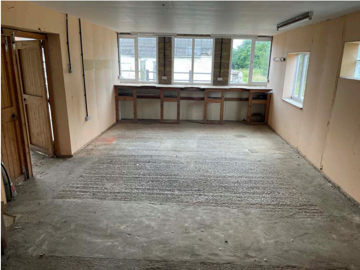
Image 14.0: Internal view of workshop/ office area.
