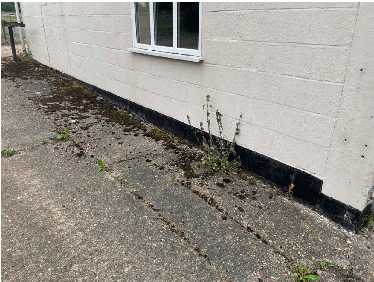
Image 3.0: Blockwork with concrete laid to falls to gable
