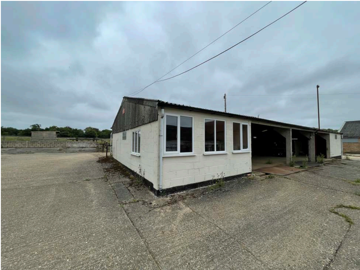
Image 1.0: View of Barn structure
