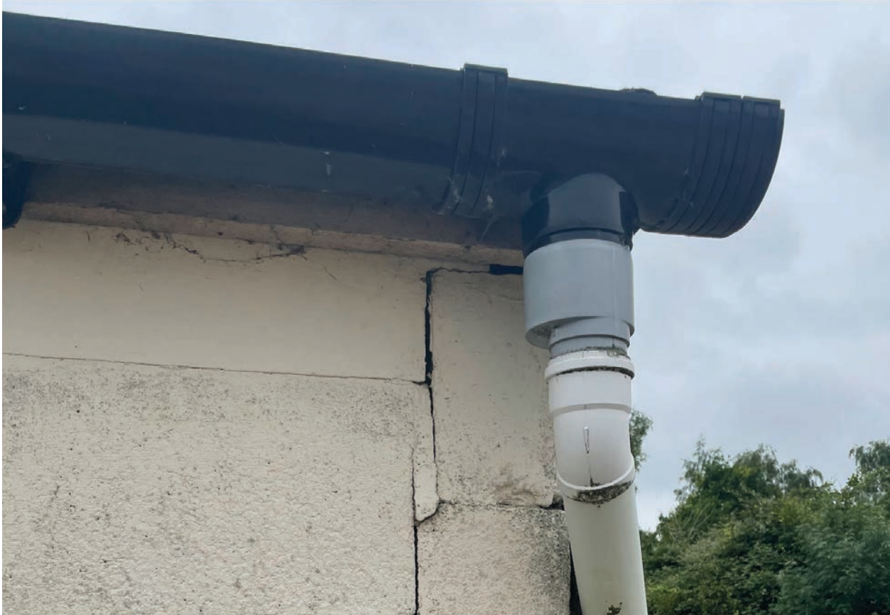
Image 12.0: Deep gutter, discharging into 75mm diameter downpipe
