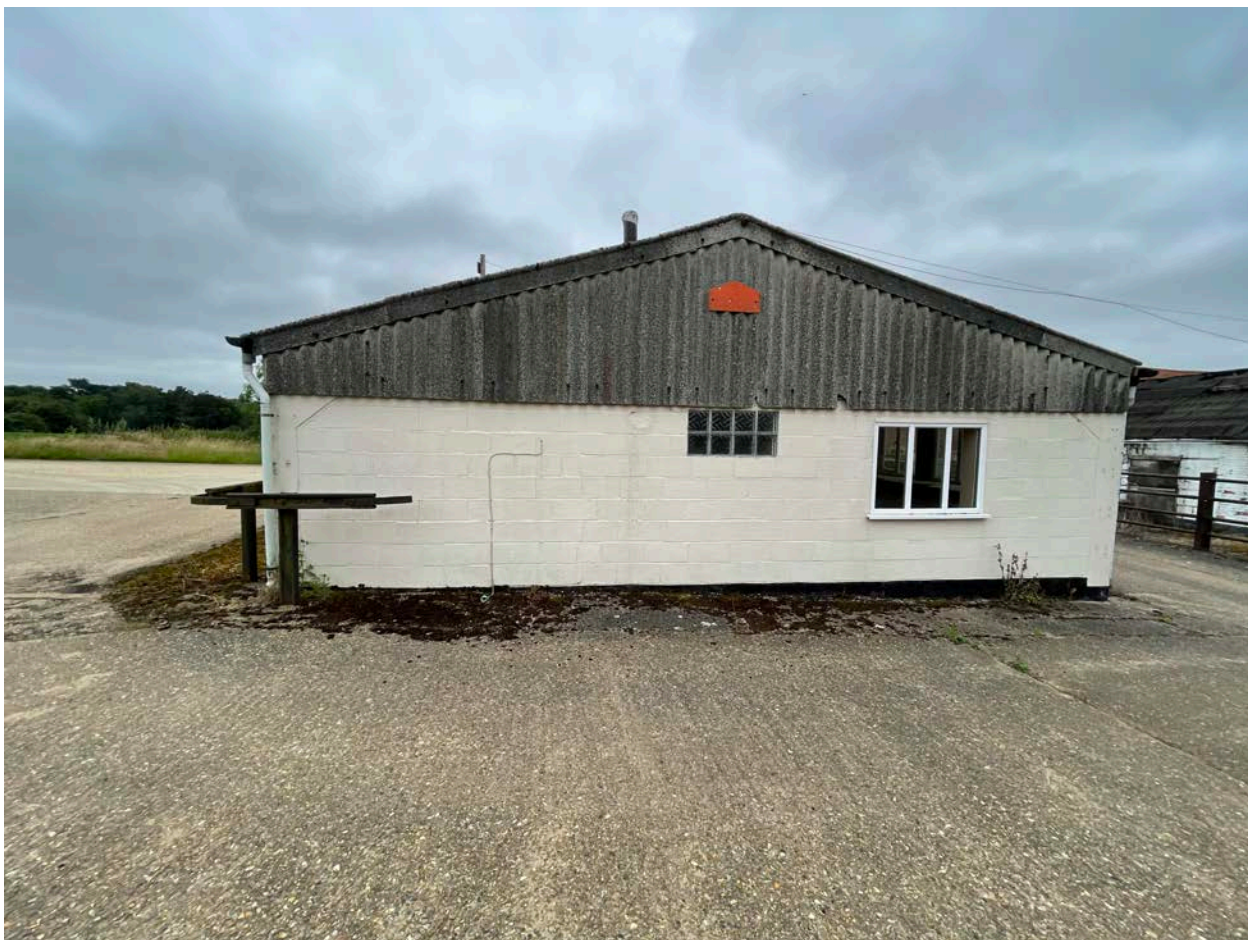
Image 2.0: Gable end to structure.
