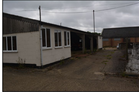
Figure 5 – View of the barn from to the south-west
