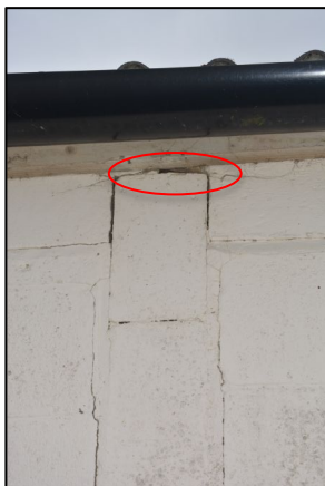
Figure 9 – Feature on the north wall pillar
