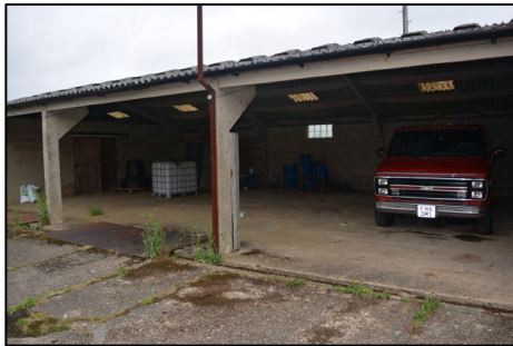
Figure 8 – View of the barn to the south
