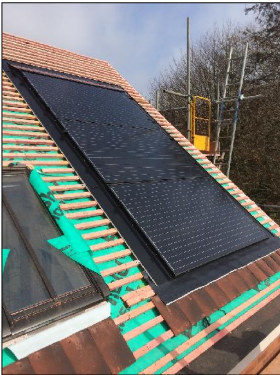
Photovoltaic Panels (in roof system)
