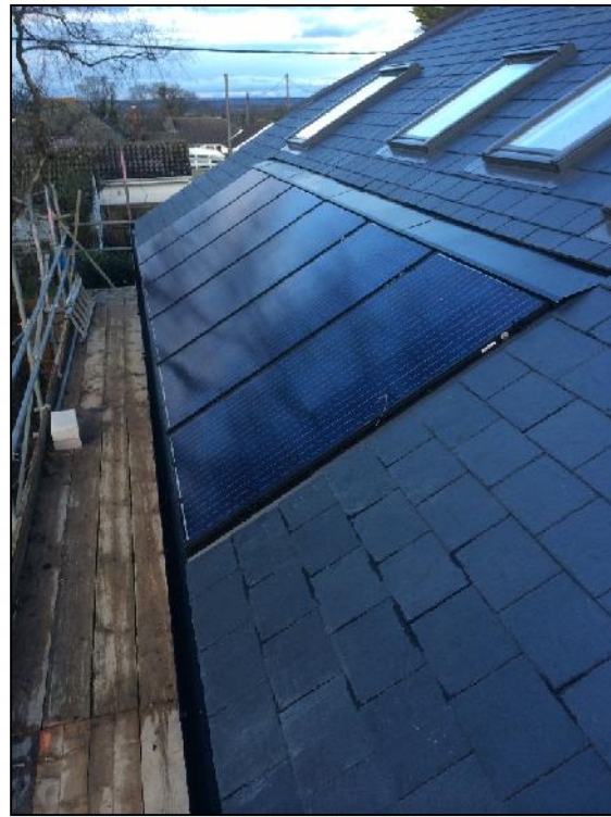
Photovoltaic Panels (in roof system)
