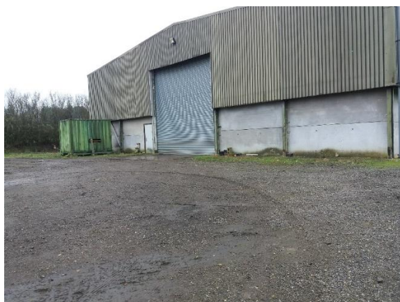
Photo 1 East elevation of the grain store
