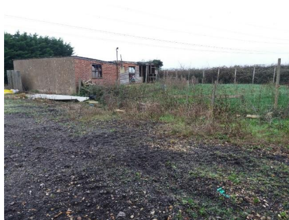
Photo 2 Stable blocks within derelict enclosure
