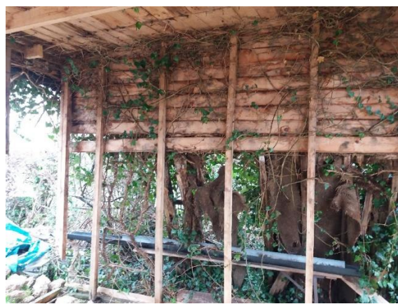
Photo 4 Interior of Block 1, with side panels removed
