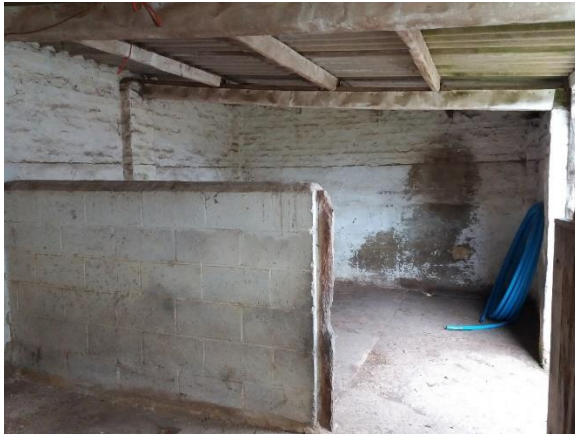
Photo 7 Interior of Block 2
