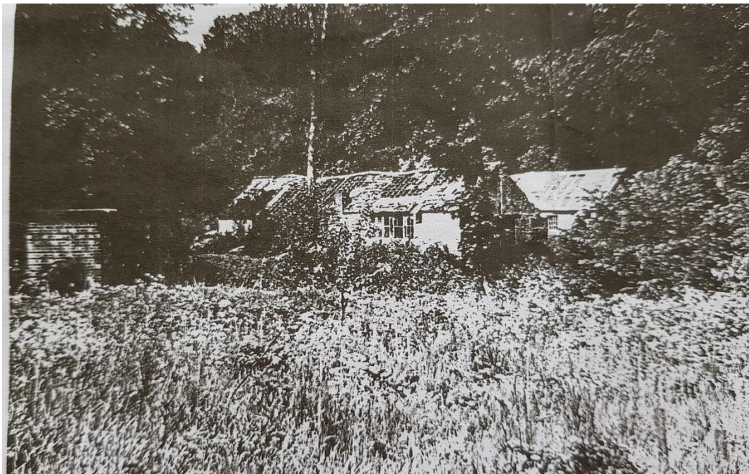
Figure 9. The site 'as existing' in 1995. The building in the foreground has mostly been demolished; only the N range survives to the rear.
