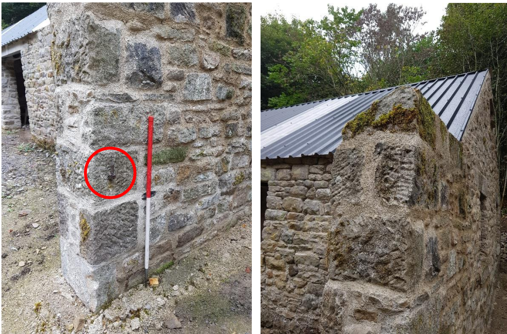
Figure 23. Left: An iron gate hinge on the E courtyard wall Right: sloping coping to the courtyard walls
