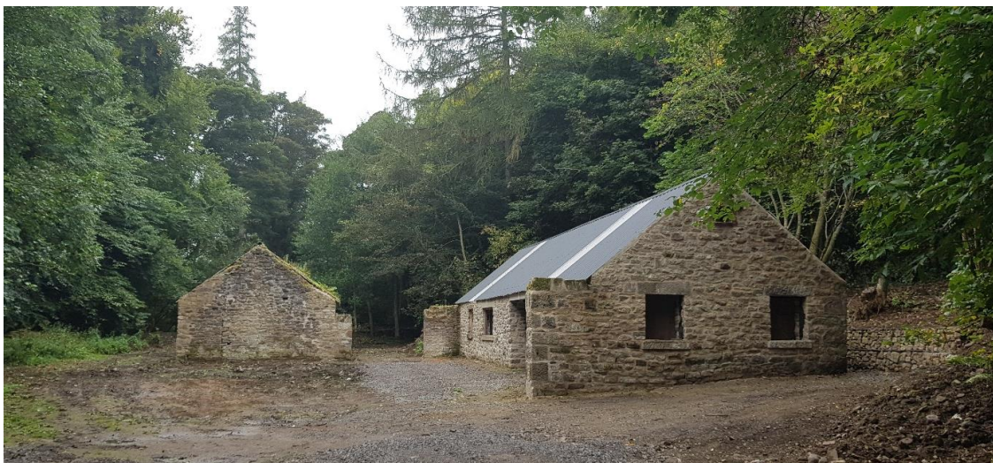
Figure 11. The site viewed from the E. The surviving range to the right is the original N range. The S range has been demolished except its W gable end. Its footprint can still be discerned on the ground. Short stretches of wall at both ends of the courtyard formed gated entrances.
