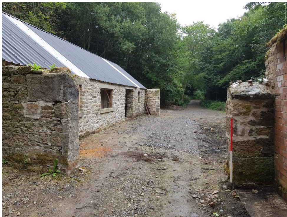
Figure 22 The three surviving courtyard walls.
