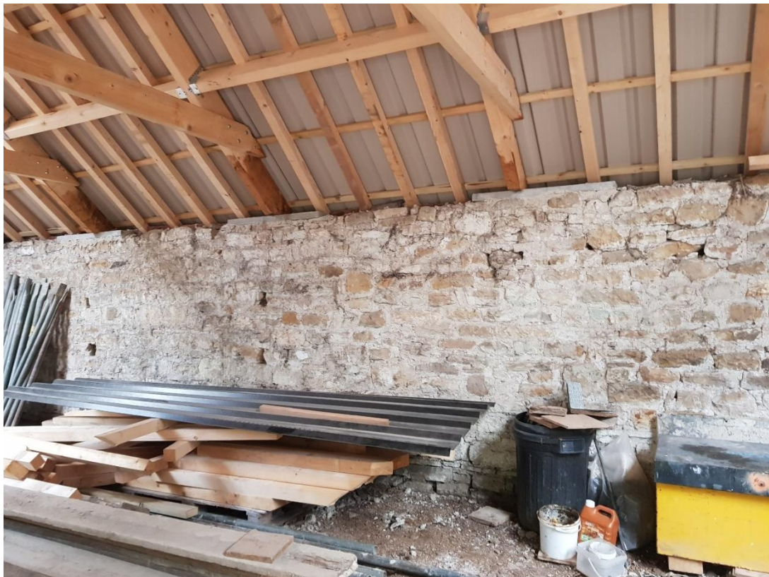
Figure 25. Plug holes on the N wall
