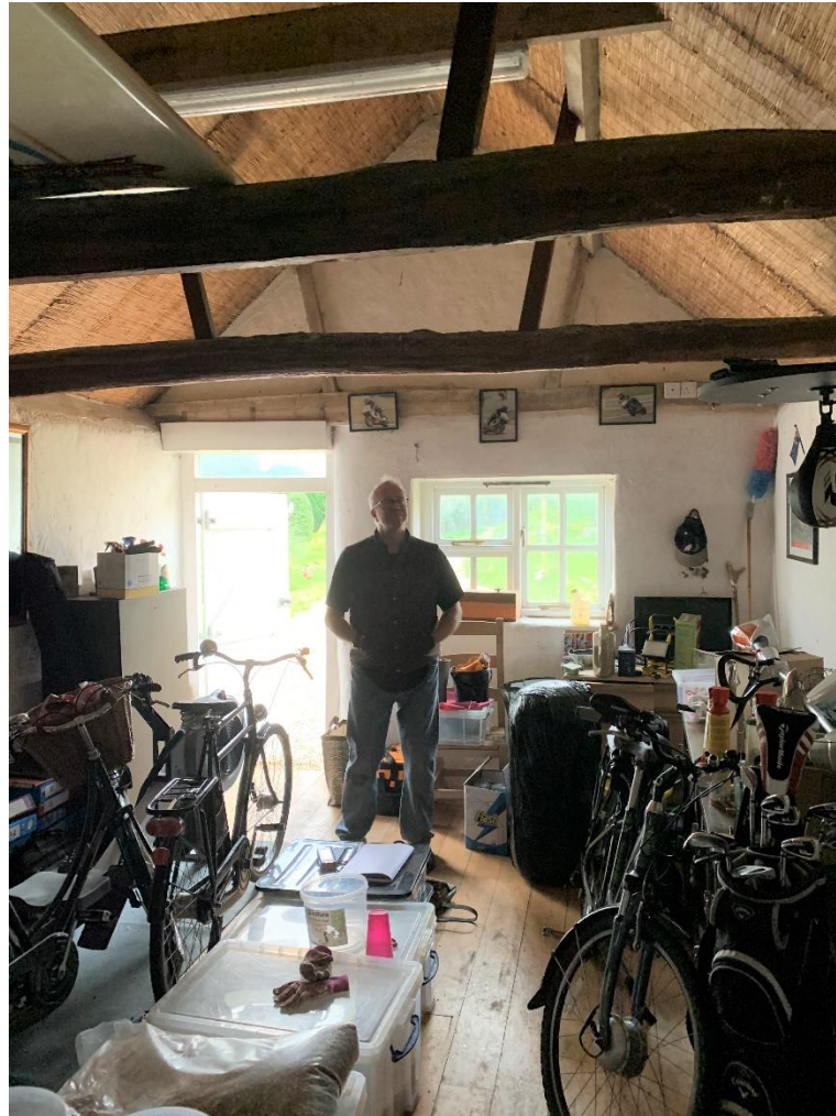
EXISTING INTERIOR OF OLD COWSHED
