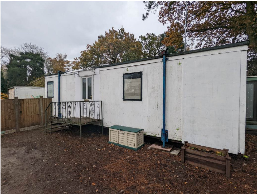
Porta cabin used for office Nov 2021
