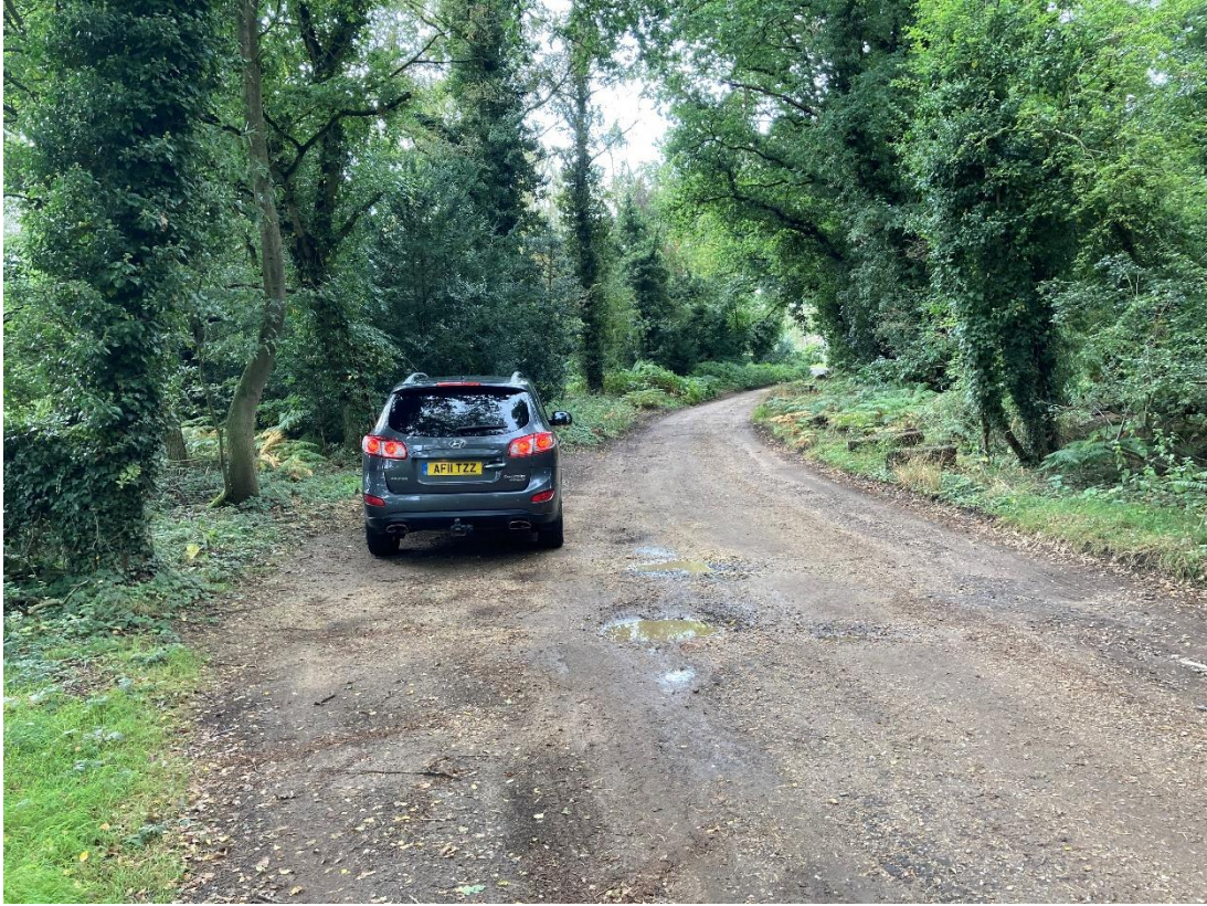
Photo 5 (Looking southbound towards the B1145)
