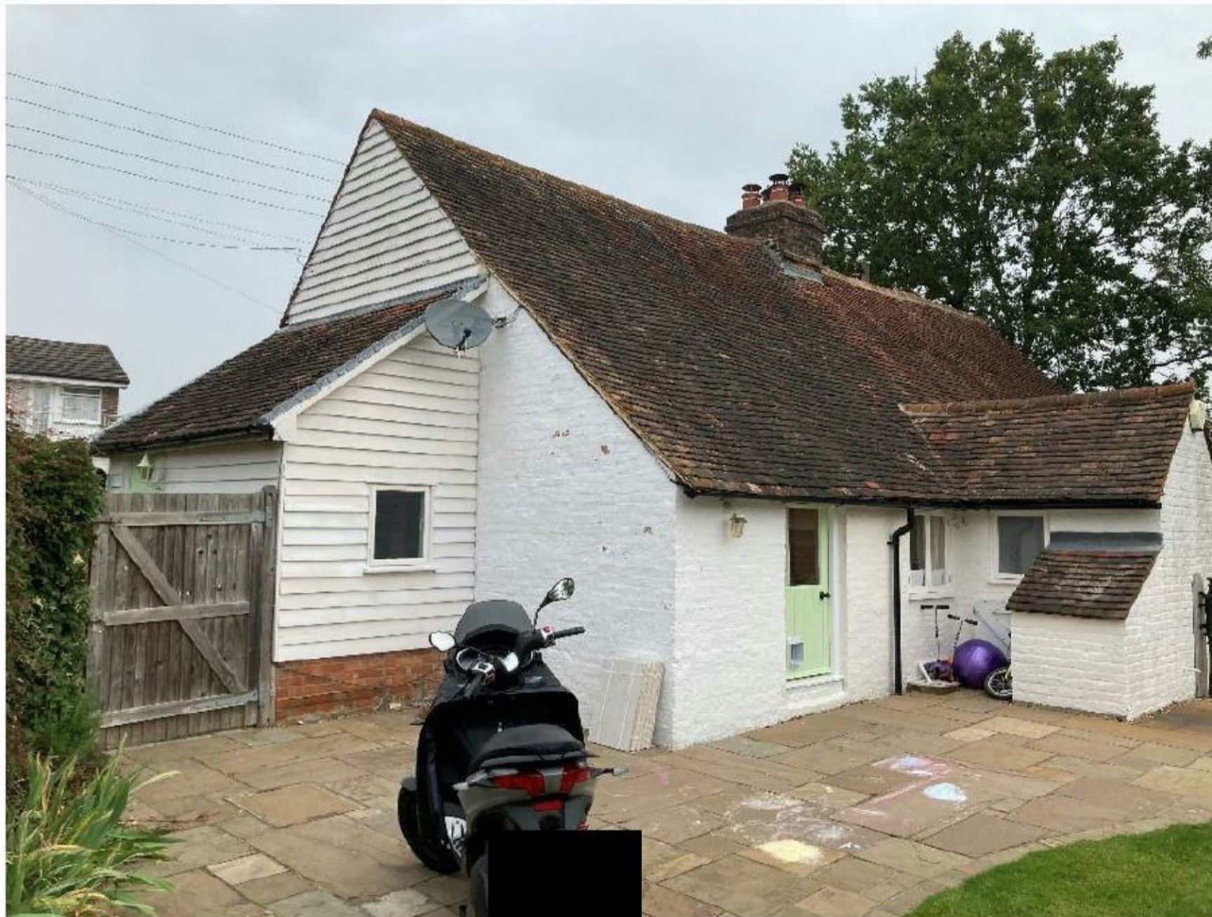
Photo of south end wall
