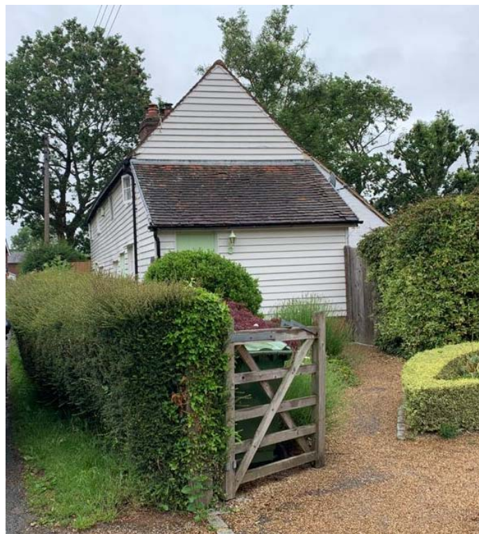
Fig 5 Photo of the existing southern gable elevation and side projection
