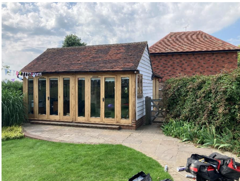
Existing outbuilding and northern flank wall of Fairview beyond
