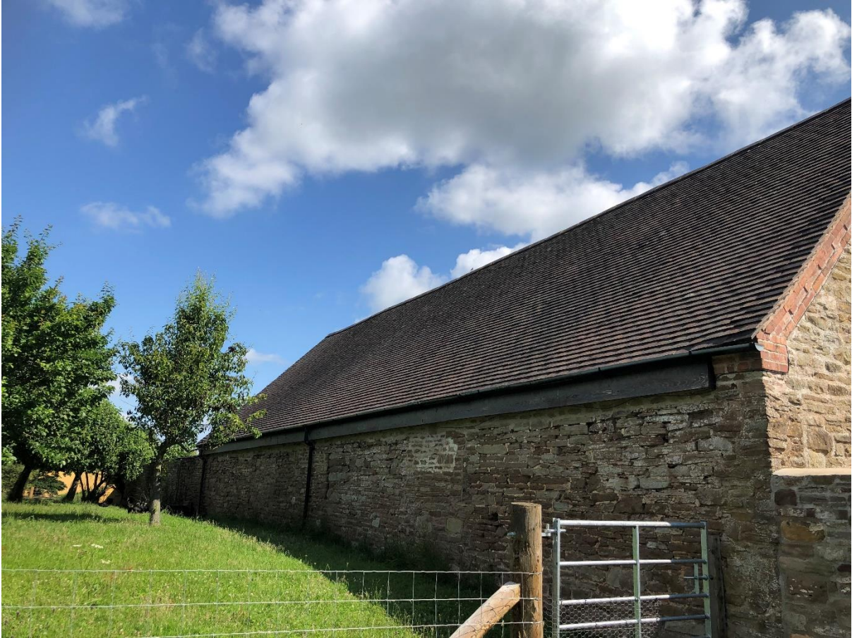
Plate 9. The rear (western) elevation of the pool house. All roof tiles are intact and this elevation offers no suitable roosting opportunities for bats.
