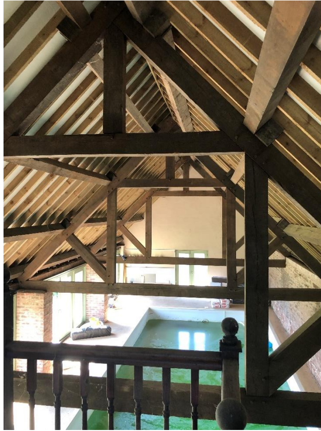
Plate 10. A view of the interior of the pool house from the mezzanine viewing platform.
