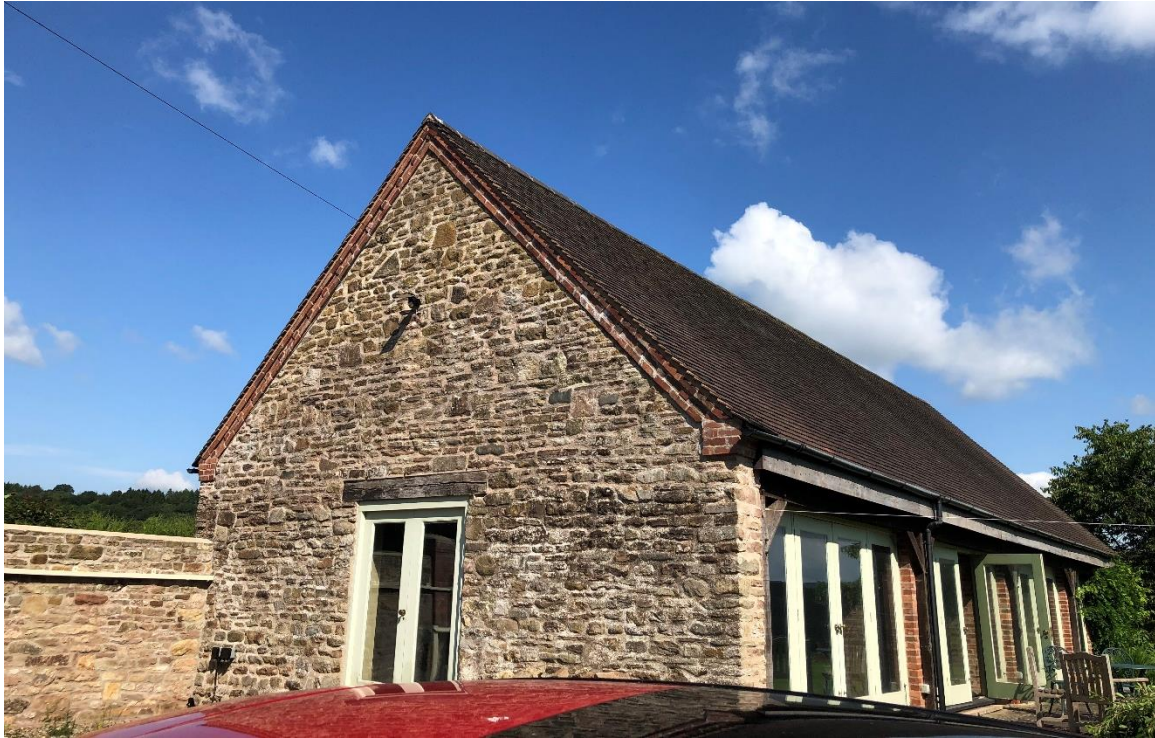
Plate 1. The southern gable end and eastern elevation of the pool house, showing stonework and roof tiles in good condition.
