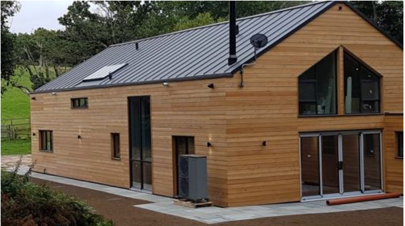
Image 3. Image of property where horizontal Siberian Larch cladding has been used to clad a new property.
